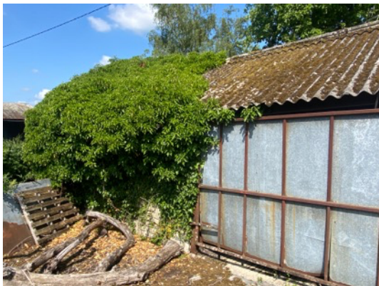
Photo 3: B1 – south-east facing elevation showing extensive ivy cover
