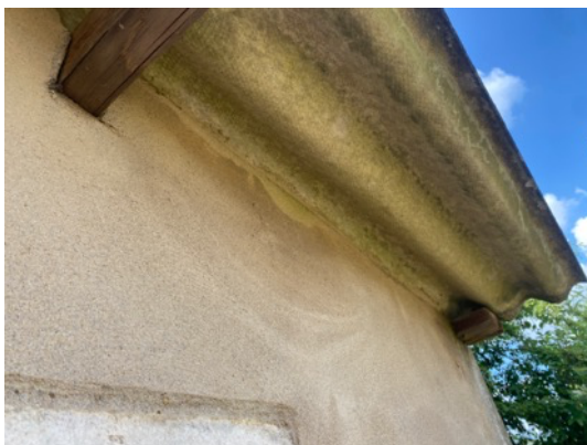
Photo 23: B5 – Roof edge without gaps or crevices suitable for roosting bats.
