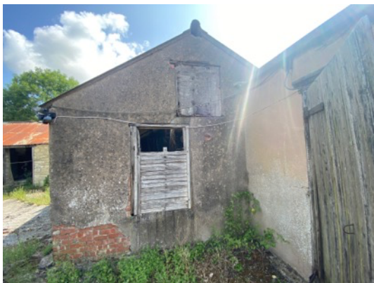
Photo 17: B4 – gap at south-eastern gable end.
