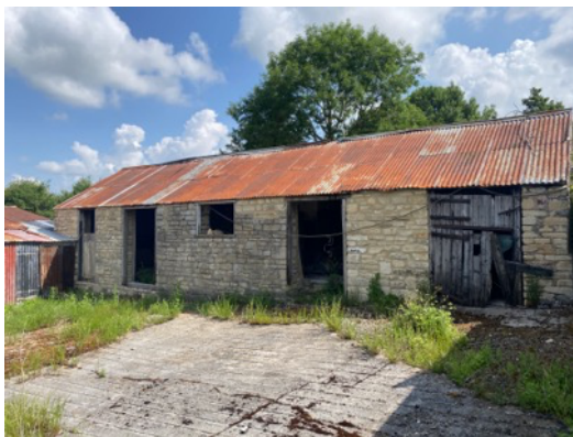
Photo 9: B3 – front south-west facing elevation showing open doorways.
