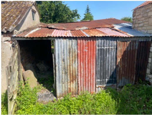
Photo 7: B2 - South-east facing elevation
