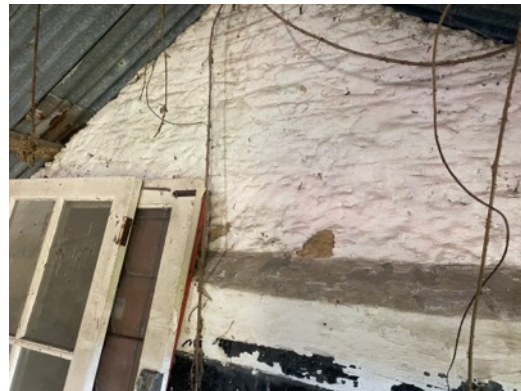
Photo 12: B3 – internal south-eastern gable end.
