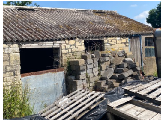
Photo 2: B1 – south-east facing elevation
