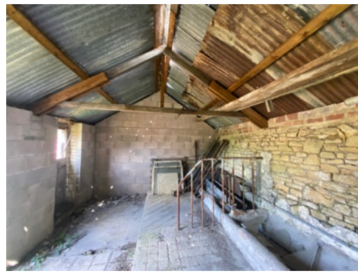
Photo 10: B3 - Internal view of roof structure.
