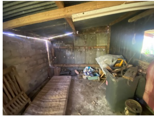
Photo 8: B2 – Internal view showing exposed timber of roof structure.
