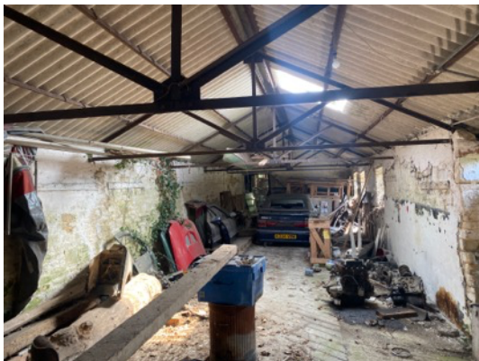
Photo 5: B1 – internal view showing skylight and metal-framed roof structure
