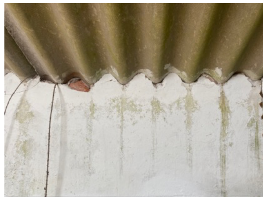
Photo 16: B4 - Internal roof edge
