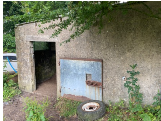
Photo 22: B5 – rear rendered concrete elevation.
