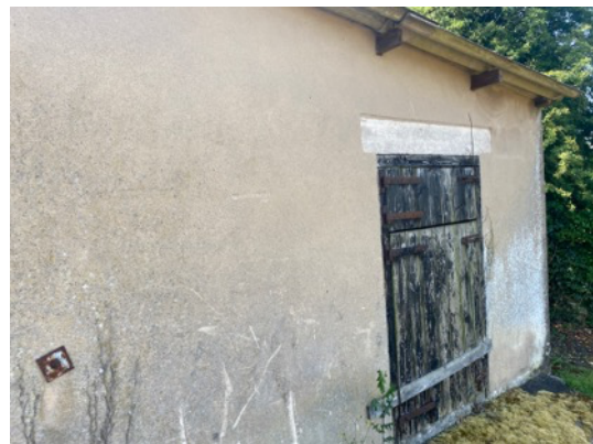
Photo 18: B5 – rendered concrete elevation
