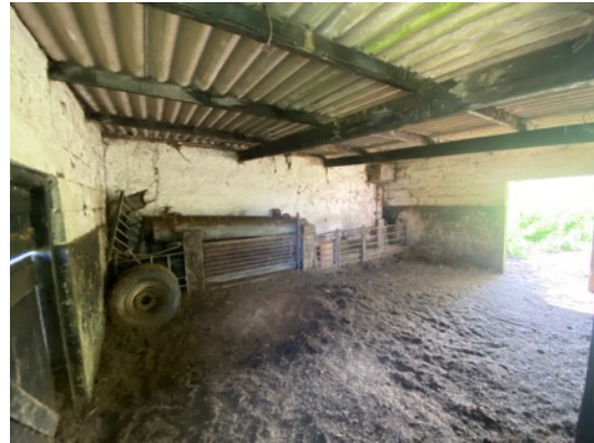
Photo 90: B5 – internal view of livestock area.
