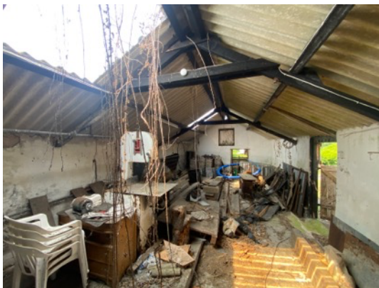
Photo 15: B4 – internal view showing skylight and exposed timber of roof structure
