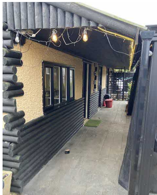
9. Looking west down the front covered path under the canopy roof.
