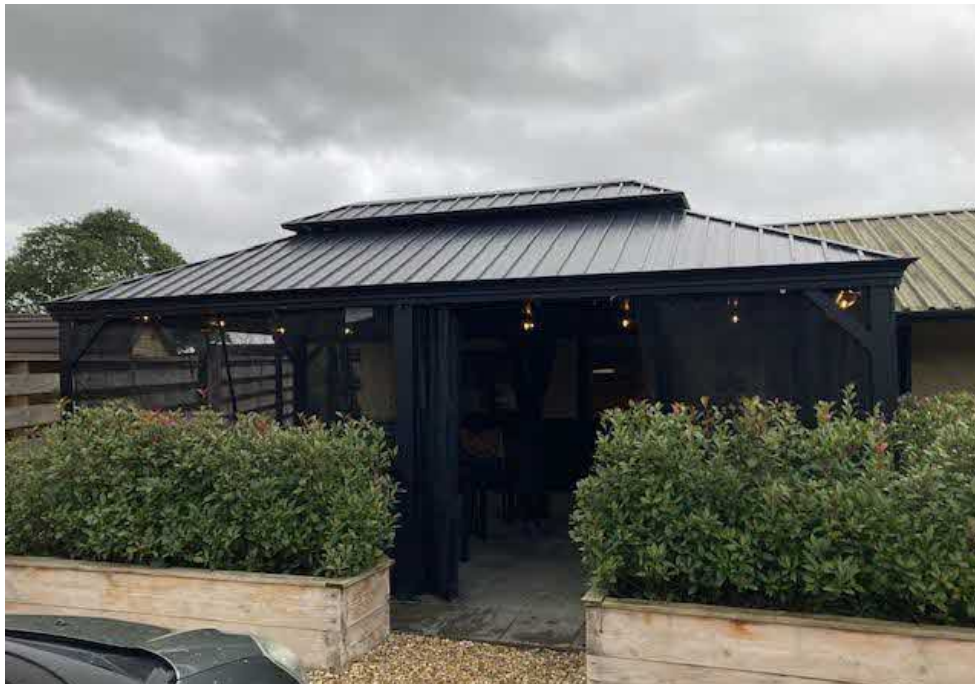
4. The pergola structure in front of the amenity building north east end.
