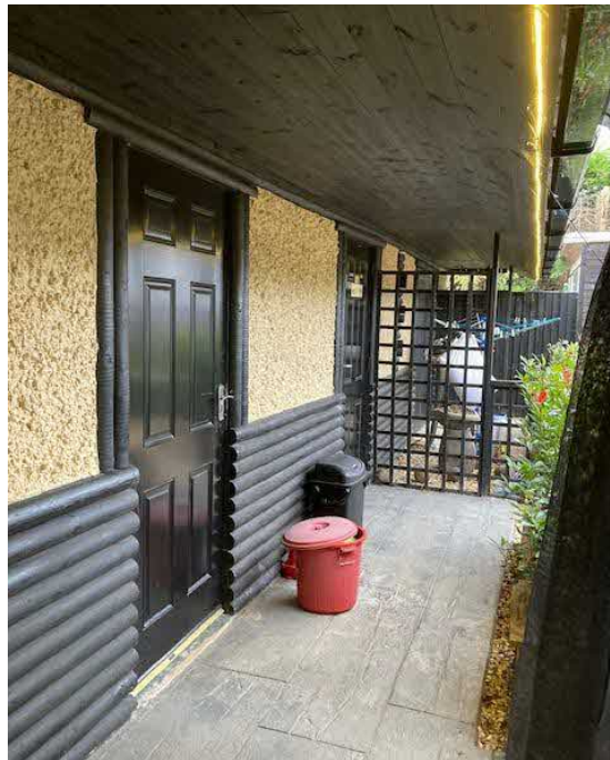
10. Looking west further under the front covered path.
