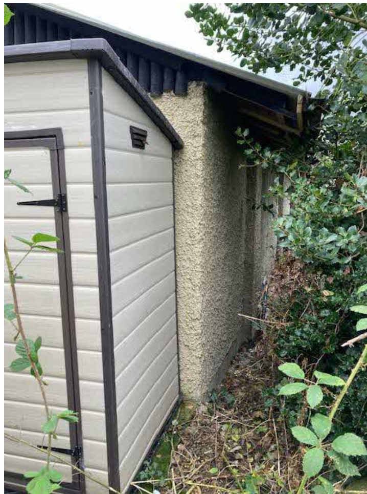
14. The rear south corner of the amenity building and small shed.
