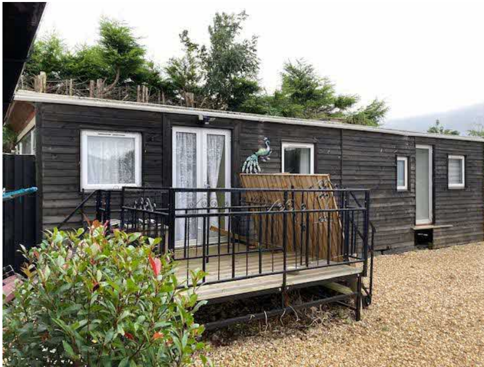
24. The front north east facing elevation of the front amenity cabin building.
