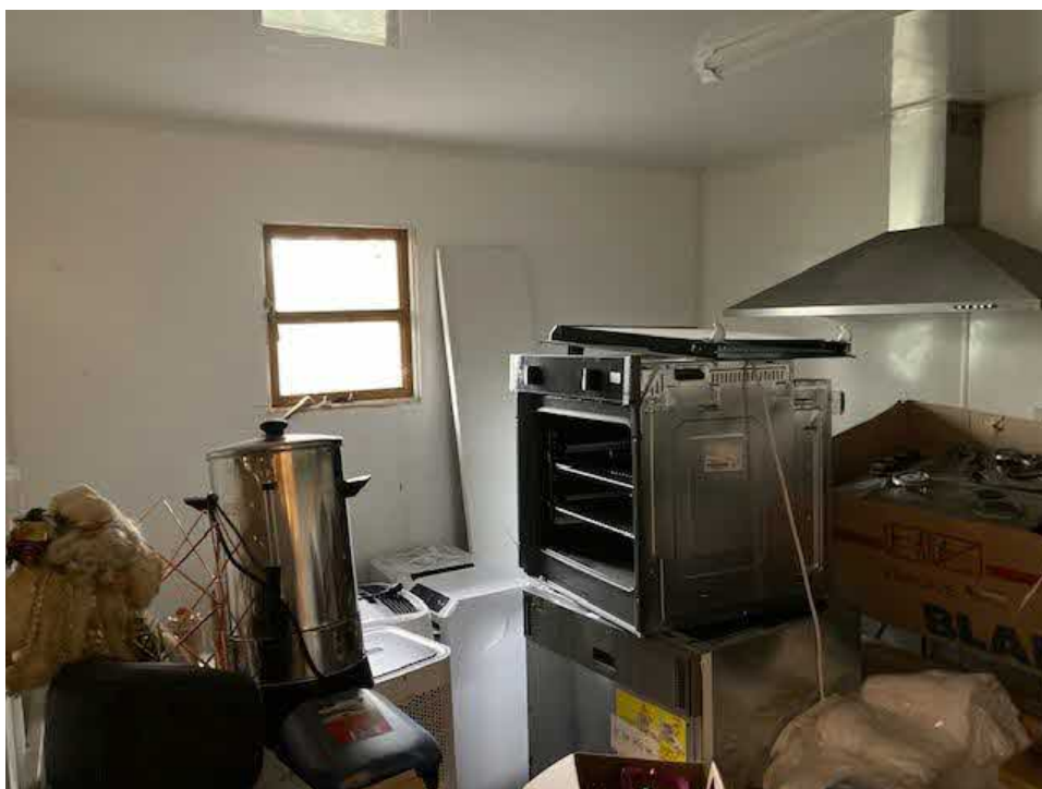
19. The kitchen (used as store room) with rear south east facing small window.
