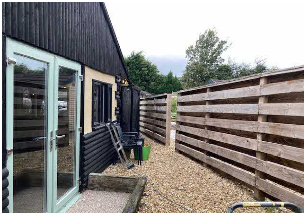
7. The timber screen fence at the north east side of the amenity building.
