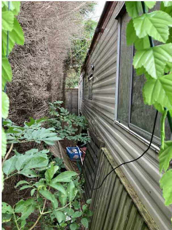
28. Looking west along the rear elevation of the cabin building.
