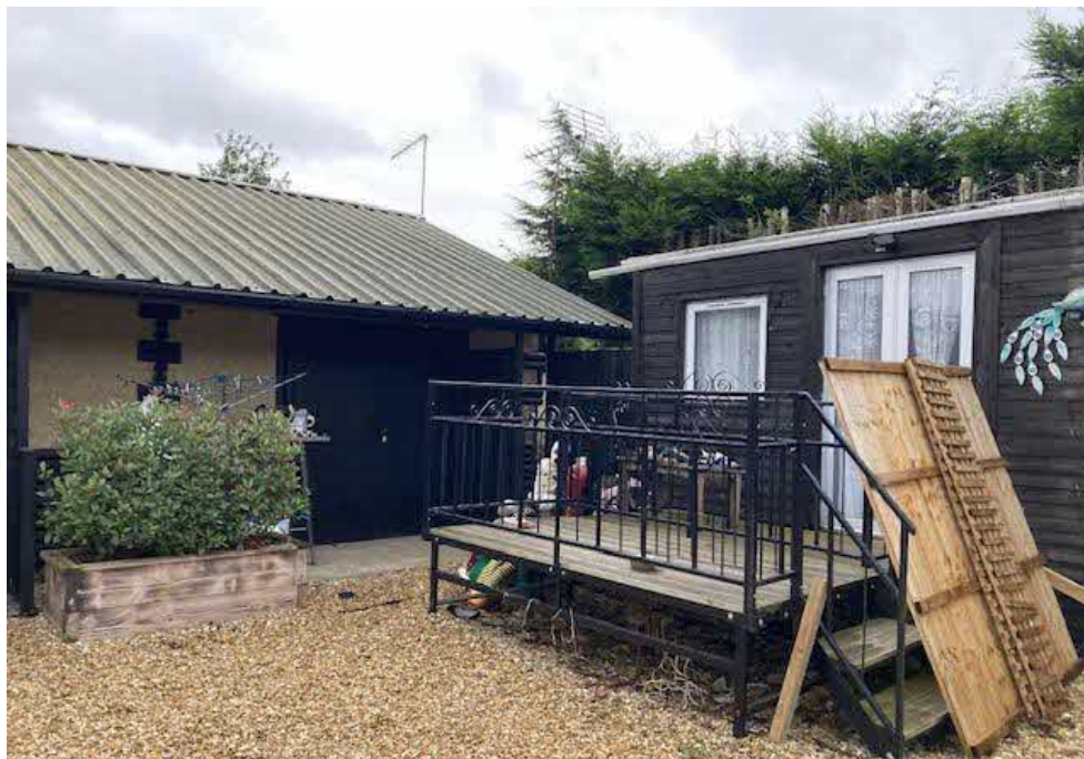
11. The south end of the amenity building adjacent to the second amenity building.
