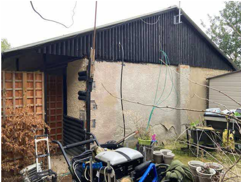
12. The south west gable end of the amenity building.
