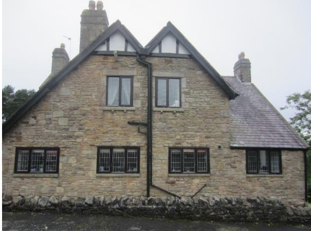
Photo 7: North-eastern elevation of the farmhouse
