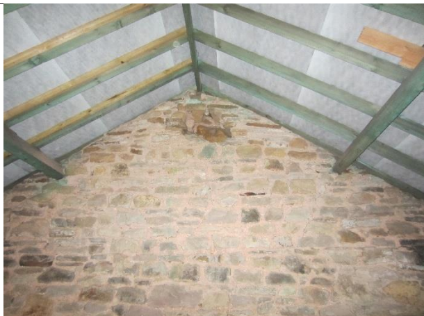
Photo 25: Underside of roof covering at Barn A
