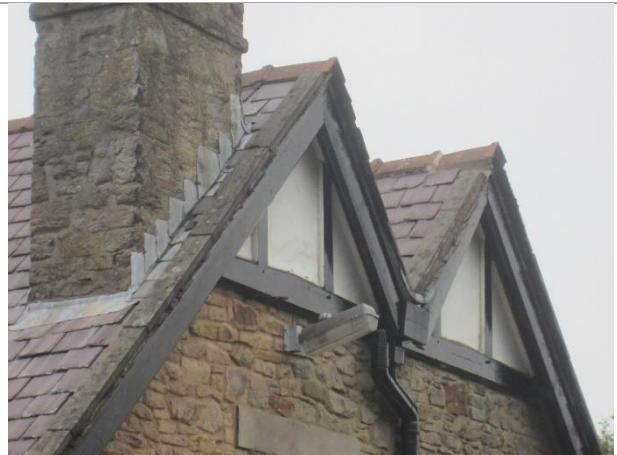
Photo 10: Timber soffits and fascia at north-eastern elevation
