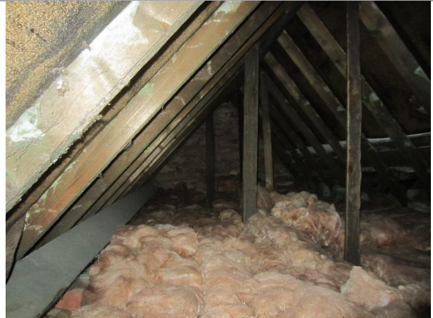
Photo 14: Roof void at farmhouse
