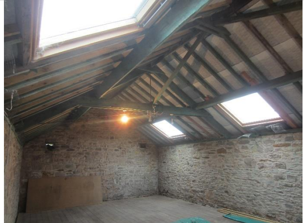
Photo 24: Interior of Barn A showing skylights and light interior
