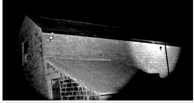
Photo 32: NVA view of Barn A
