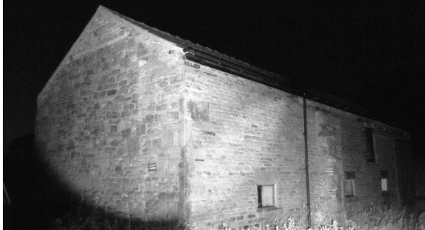
Photo 33: NVA view of Barn A
