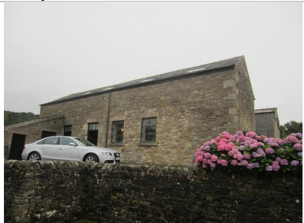
Photo 18: North-western elevation of Barn A
