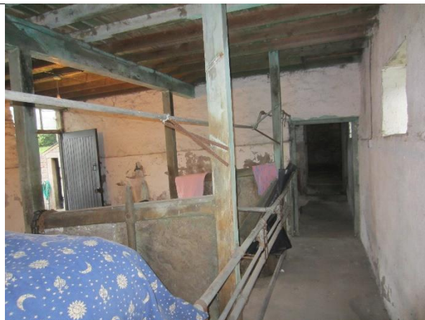
Photo 26: Interior of Barn A (ground floor)
