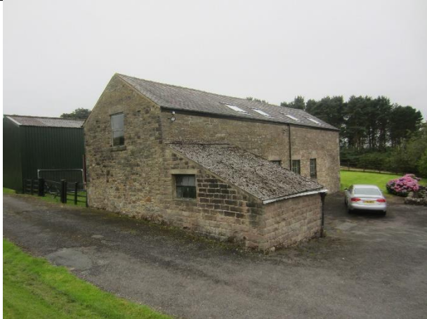
Photo 19: North-eastern and north-western elevations of Barn A
