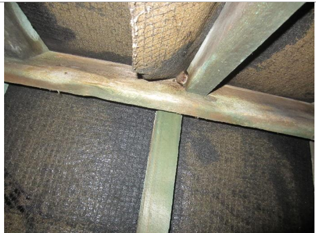
Photo 16: Brown long-eared bat in roof void at farmhouse [Roost D]
