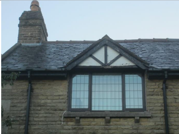
Photo 13: South-western elevation of the farmhouse
