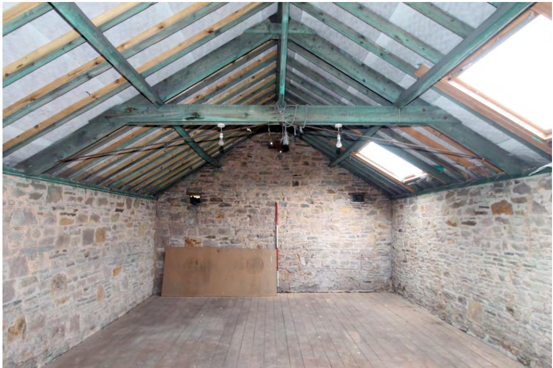
Plate 29. Barn, hayloft, viewed from north-east.
