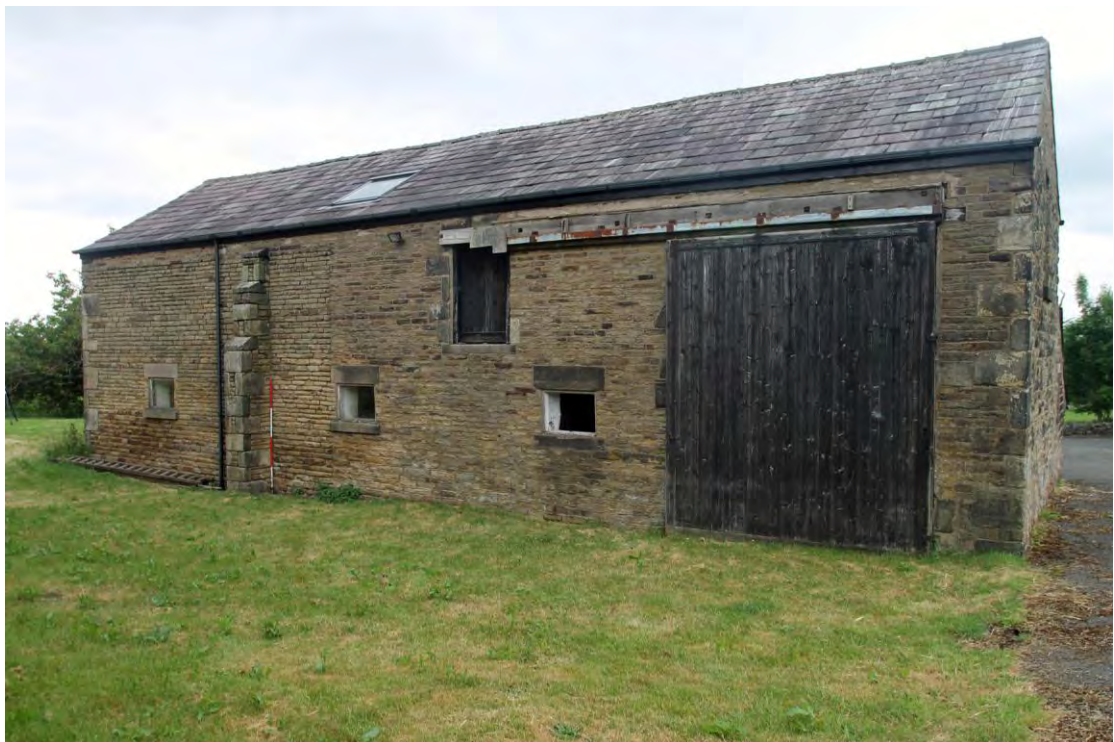
Plate 4. Barn south elevation, viewed from south-east.
