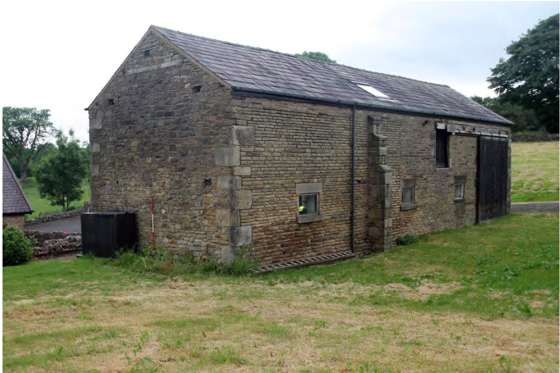
Plate 3. Barn south elevation, viewed from south-west.
