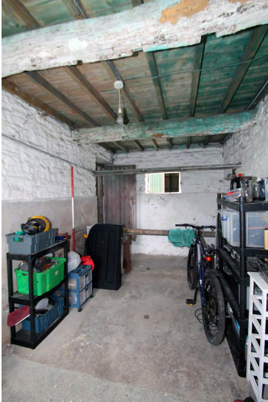
Plate 18. Barn, room G2, viewed from north-west.
