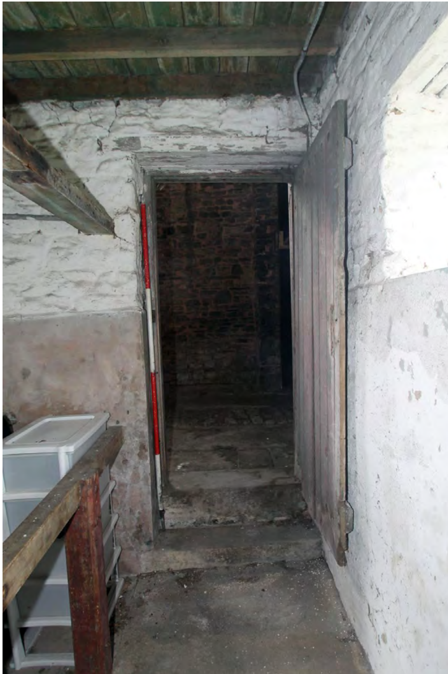
Plate 20. Barn, room G2, feed passage, viewed from south-west.
