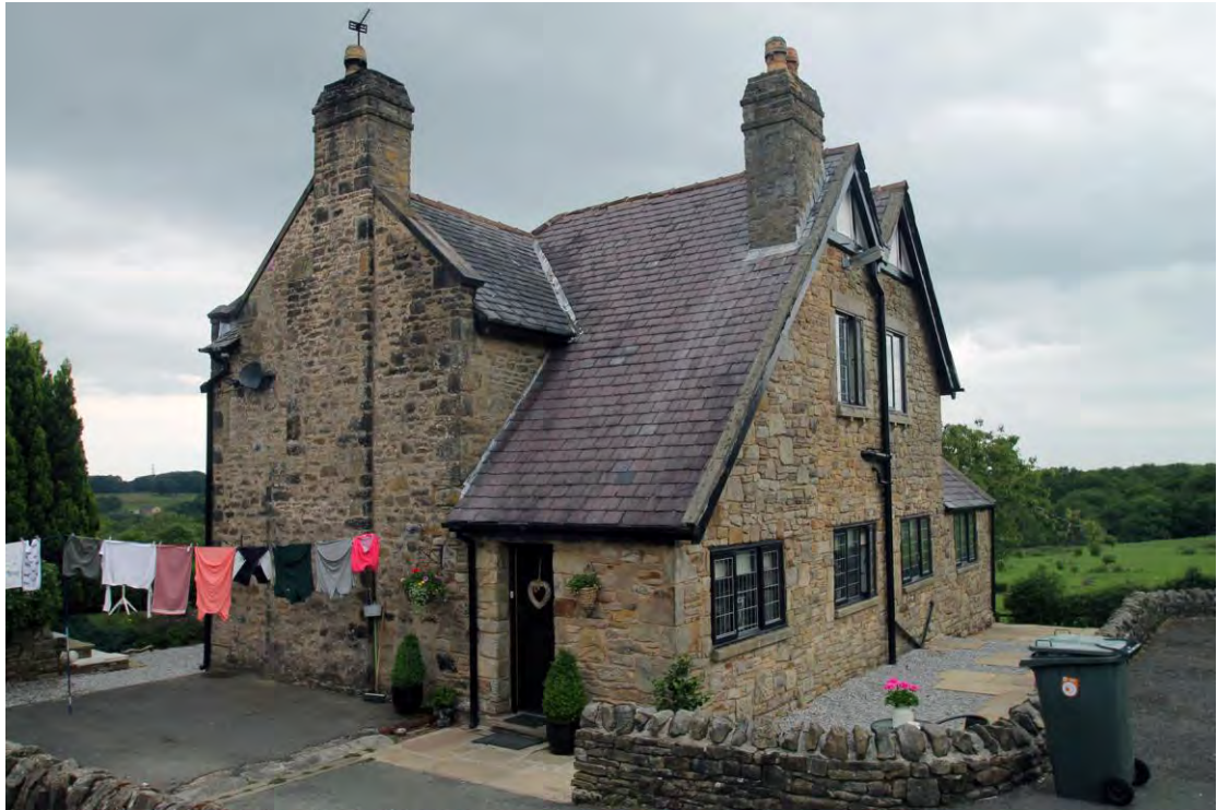
Plate 32. Farmhouse, viewed from south-east.
