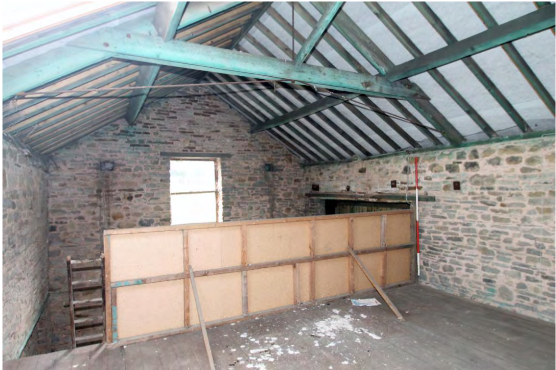
Plate 26. Barn, hayloft, viewed from south-west.
