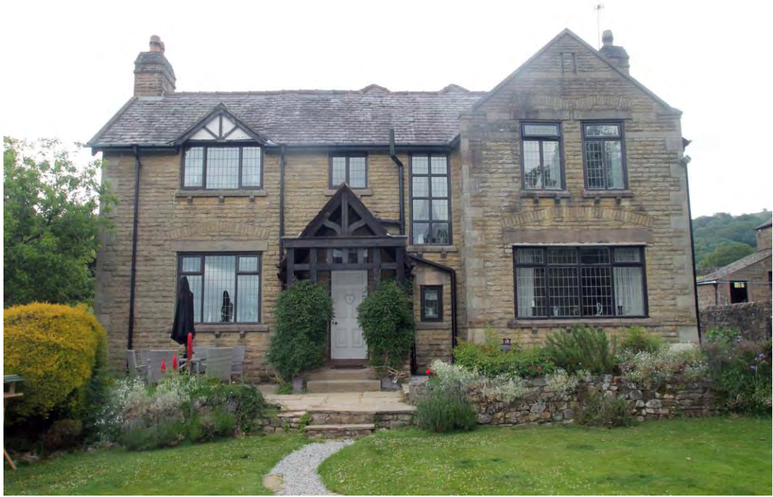
Plate 30. Farmhouse, viewed from south-west.
