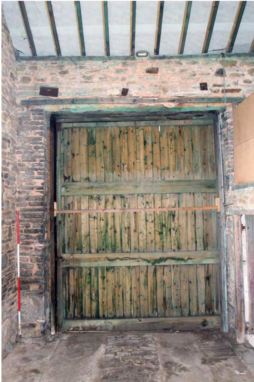
Plate 22. Barn, room G3, viewed from north-east.
