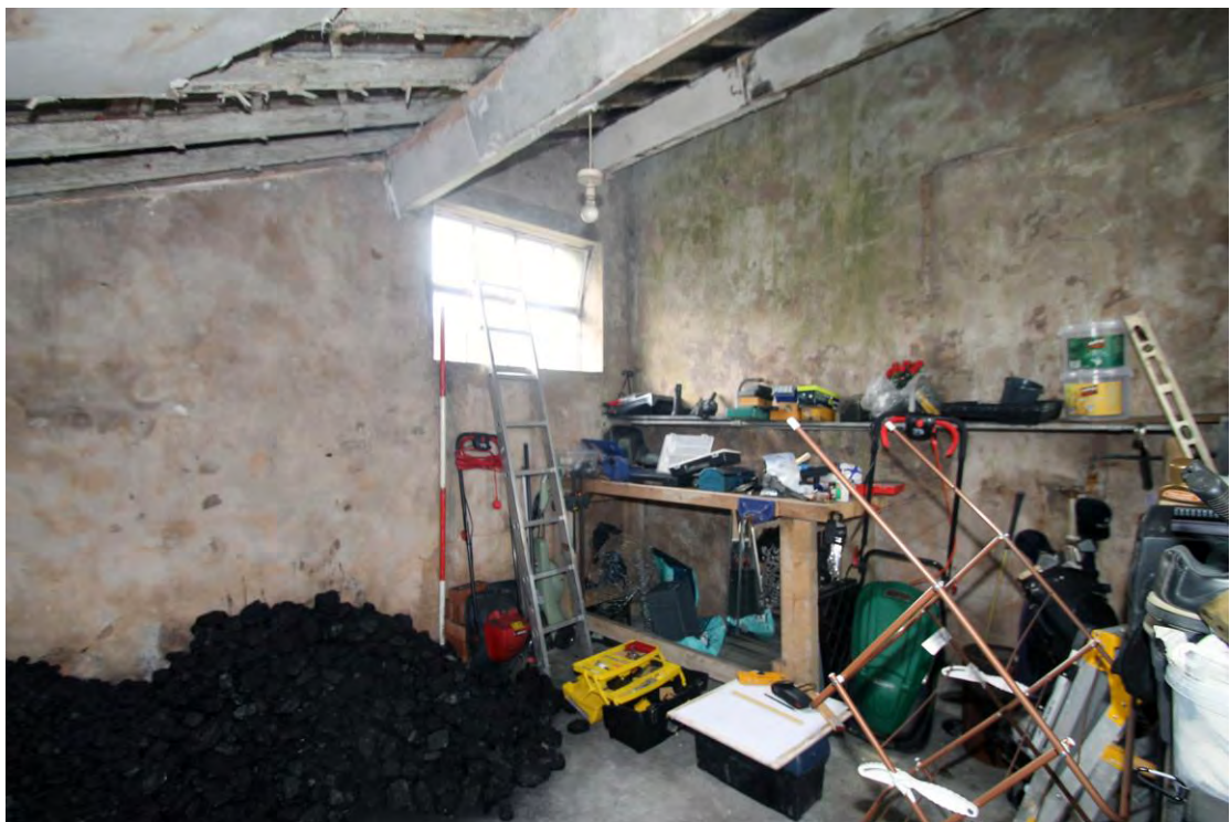
Plate 24. Barn, room G4, viewed from west.
