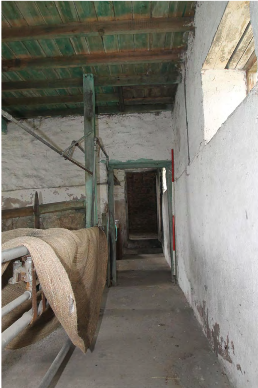
Plate 16. Barn, room G1, view along feed passage, from south-west.
