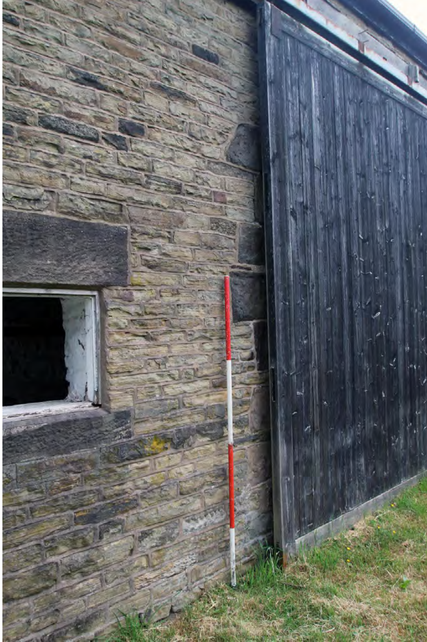
Plate 6. Doorway to drift house, in barn south elevation, viewed from south-west.
