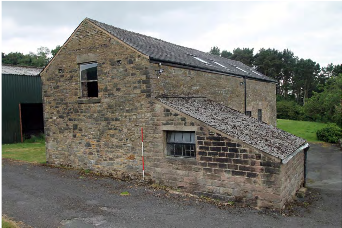
Plate 10. Barn, east elevation, viewed from north-east.
