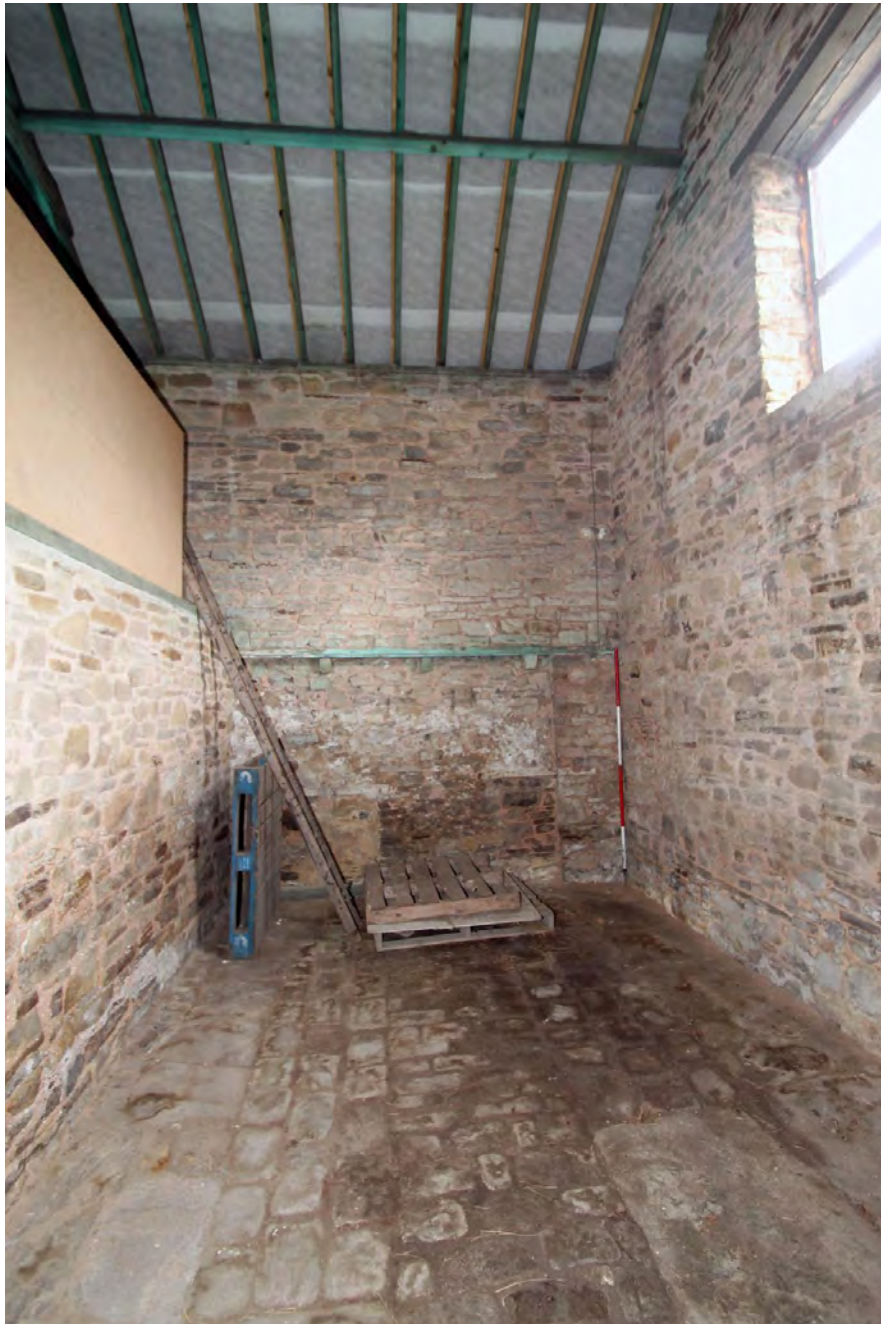
Plate 21. Barn, room G3, viewed from south-east.
