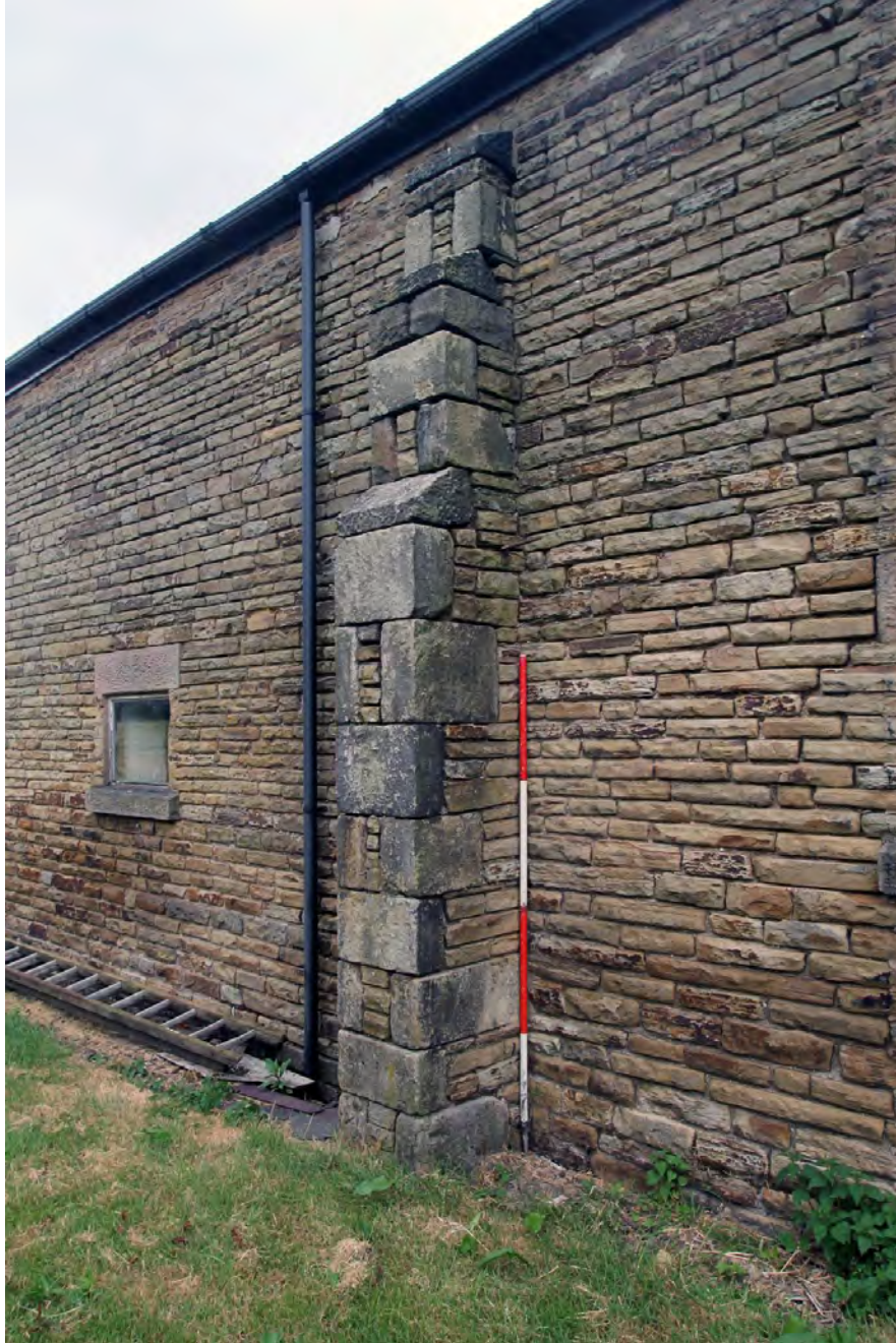
Plate 5. Buttress in barn south elevation, viewed from east.
