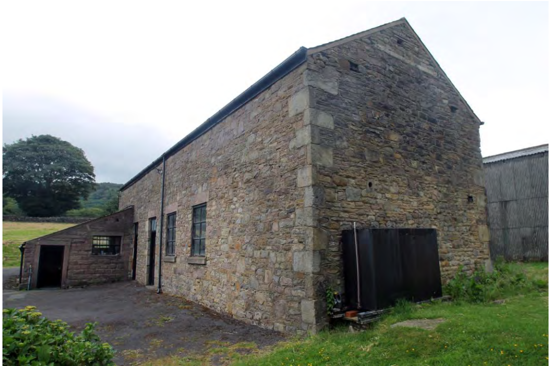
Plate 12. Barn, viewed from west.
