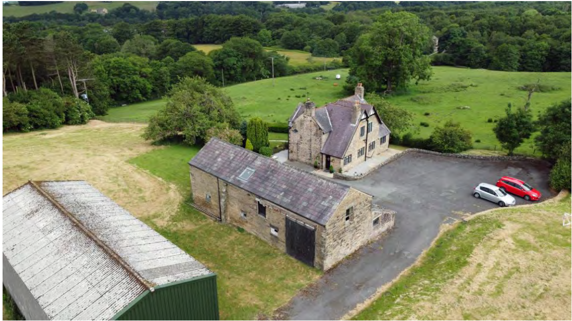
Plate 1. Site viewed from east, barn in centre.
