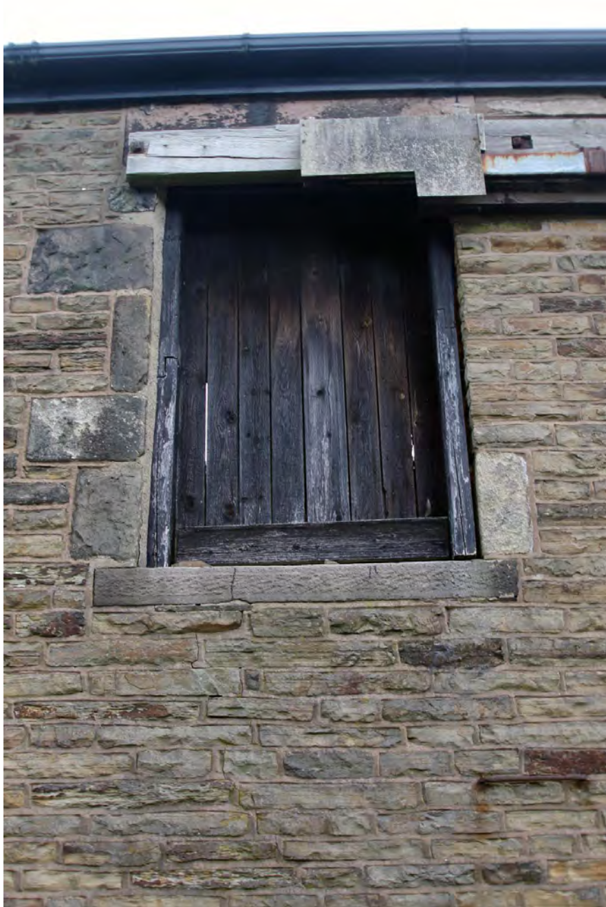
Plate 7. Taking in door in barn south elevation, viewed from south.
