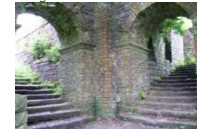
2. Archways to Rivington Gardens
