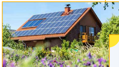
Photovoltaic thermal (PVT)
