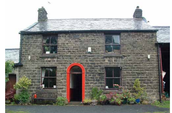
Middle Derbyshire Farm - Former Structure (Now Demolished) - Image 2
