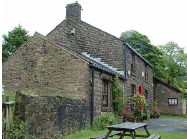
Middle Derbyshire Farm - Former Structure (Now Demolished) - Image 1
