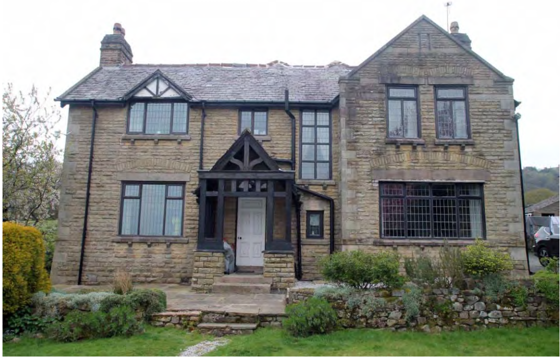
Plate 1. West elevation, viewed from west.
