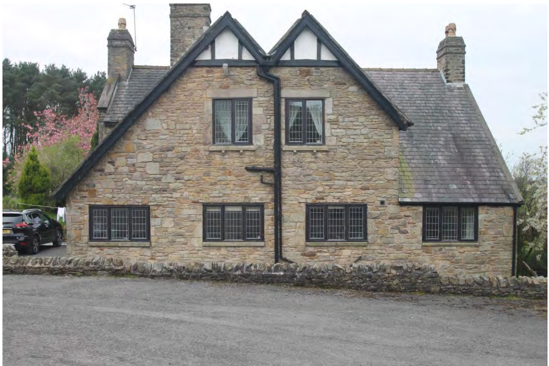
Plate 6. East elevation, viewed from east.
