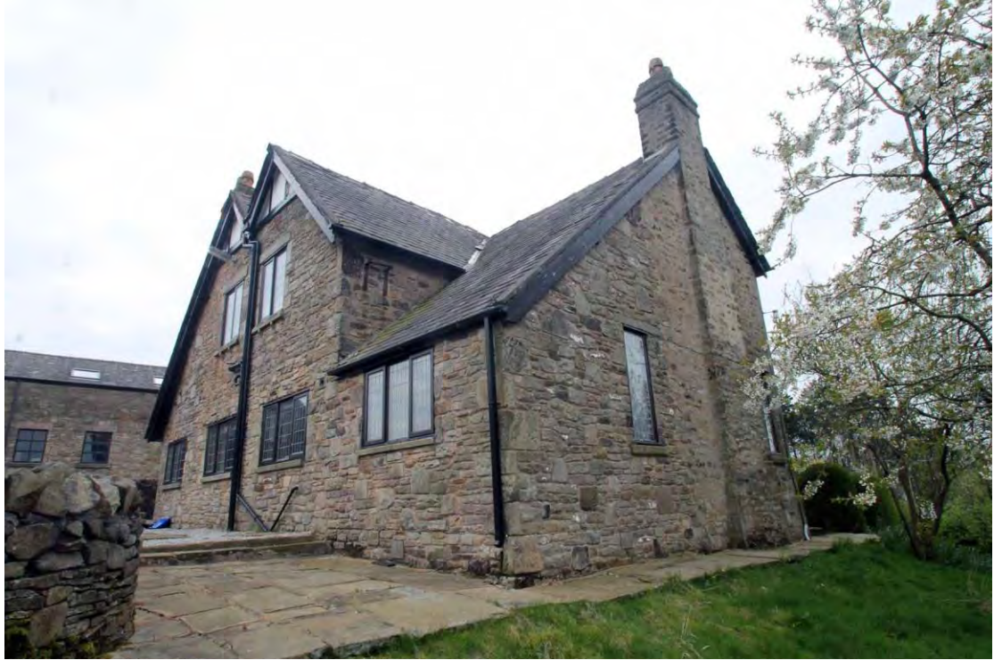
Plate 7. East and north elevations, viewed from north-east.
