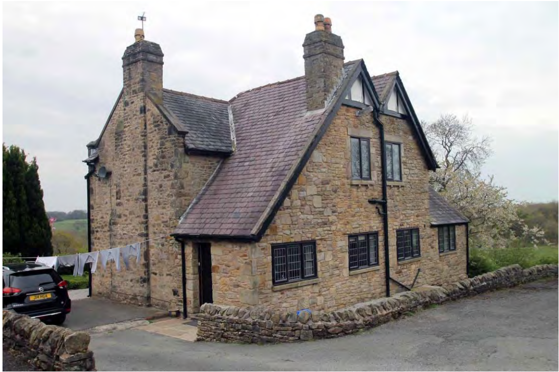
Plate 5. South and east elevations, viewed from south-east.
