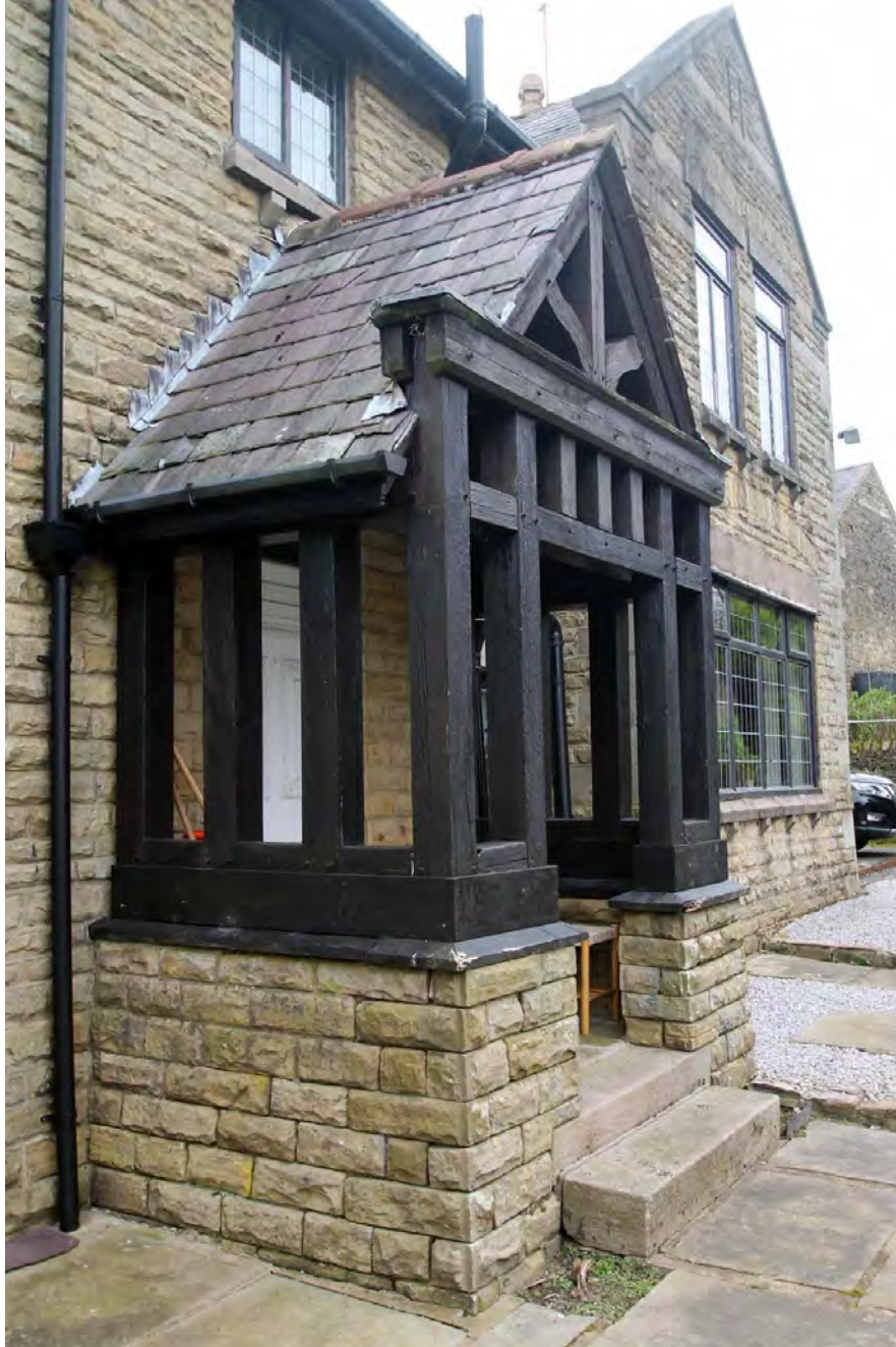
Plate 3. External porch, viewed from north-west.
