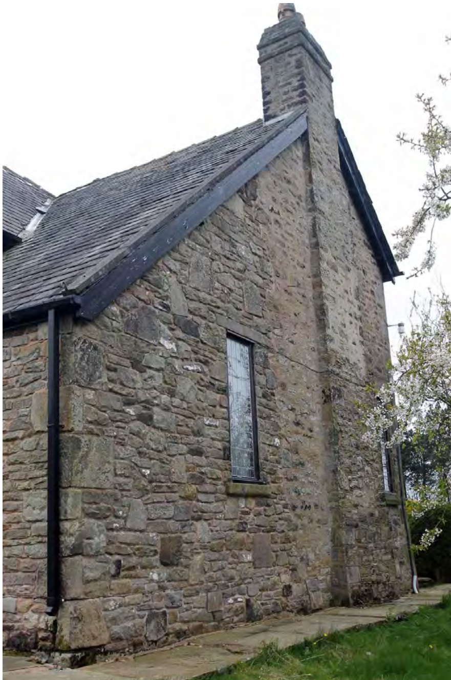
Plate 8. North elevation, viewed from north-east.
