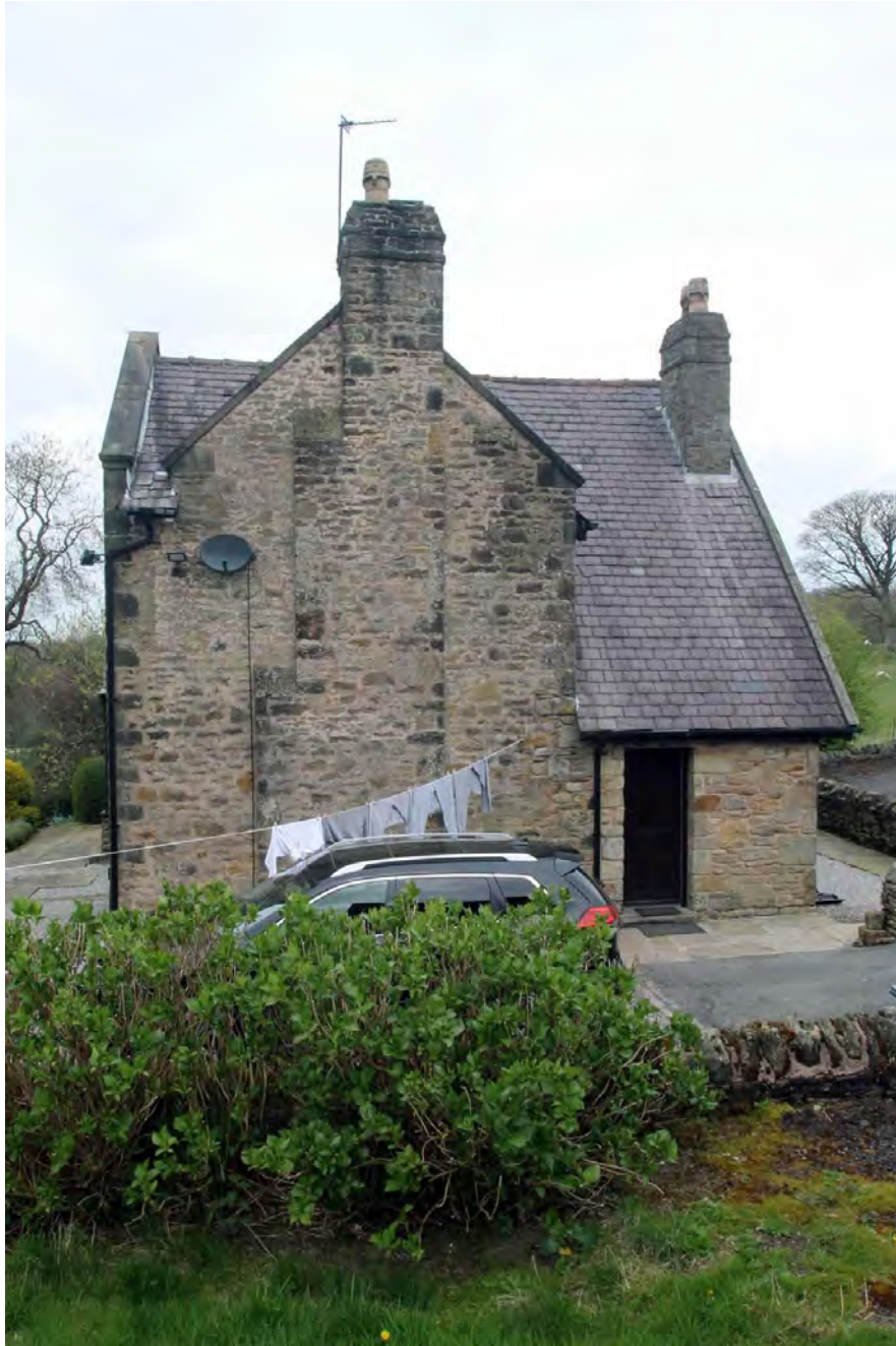
Plate 4. South elevation, viewed from south.
