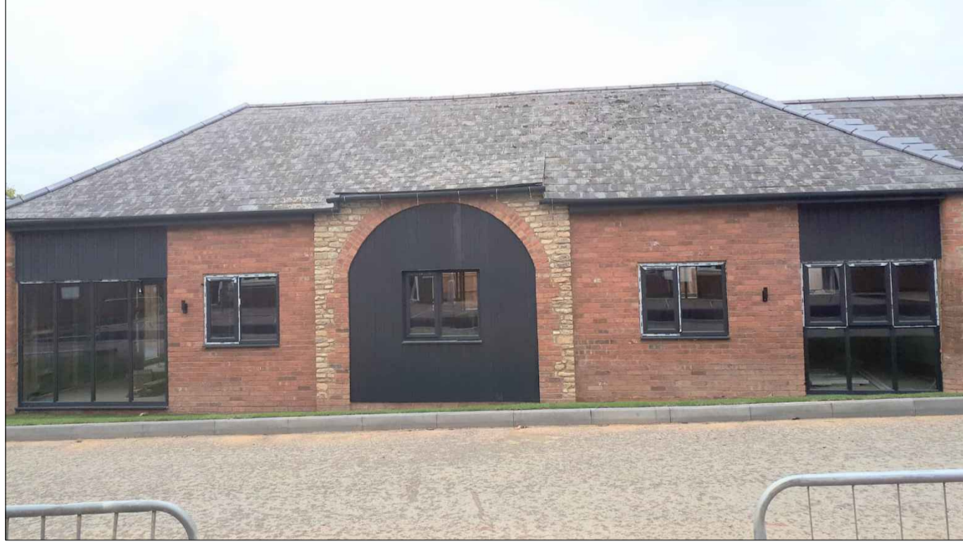
Photo of rebuilt section of wall
