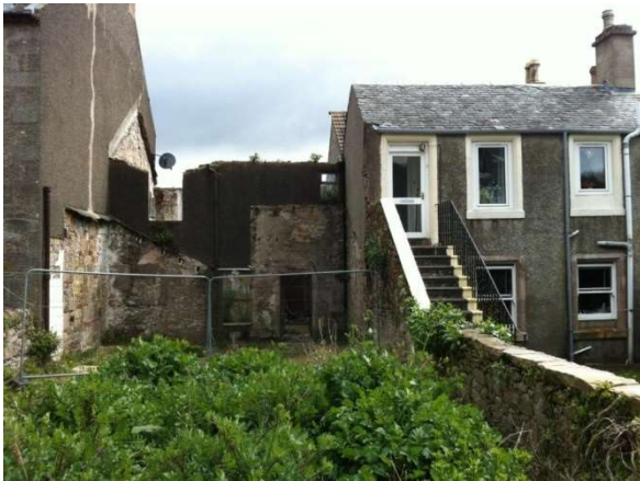
Looking into the rear of the site
