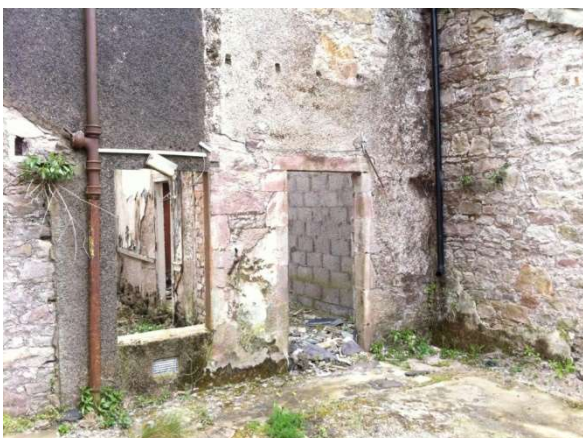
Rear walling to house fronting Crichton Street
