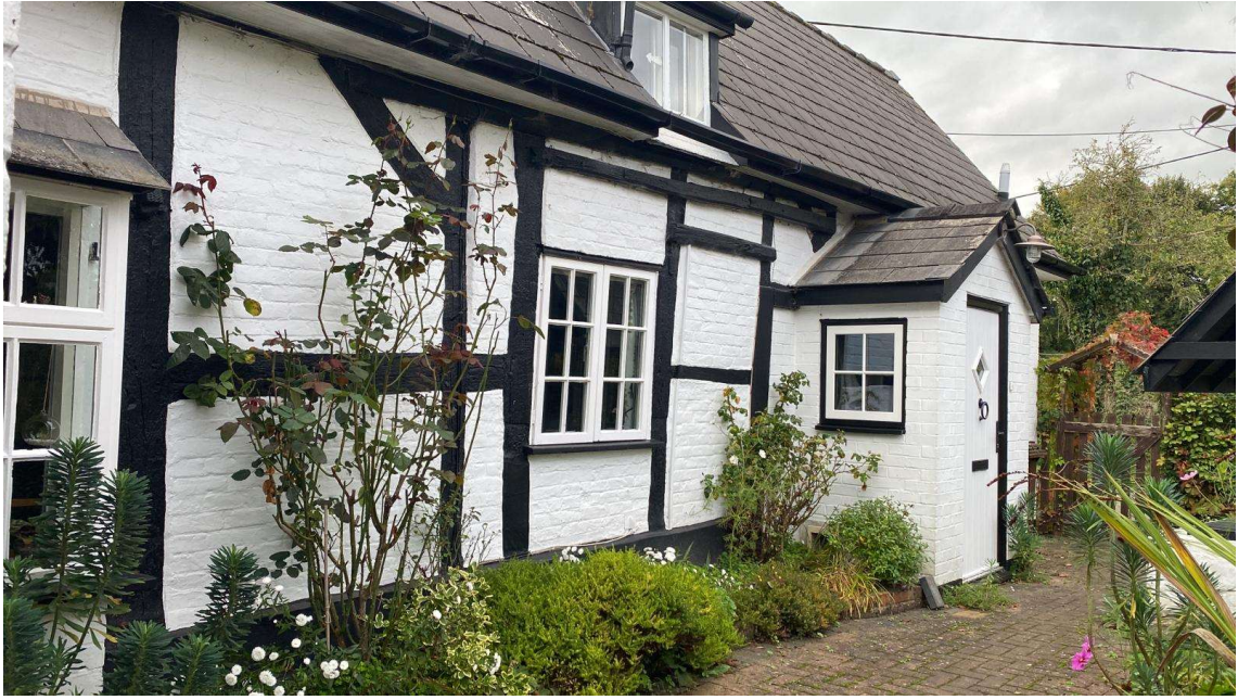
The Front Porch before works
