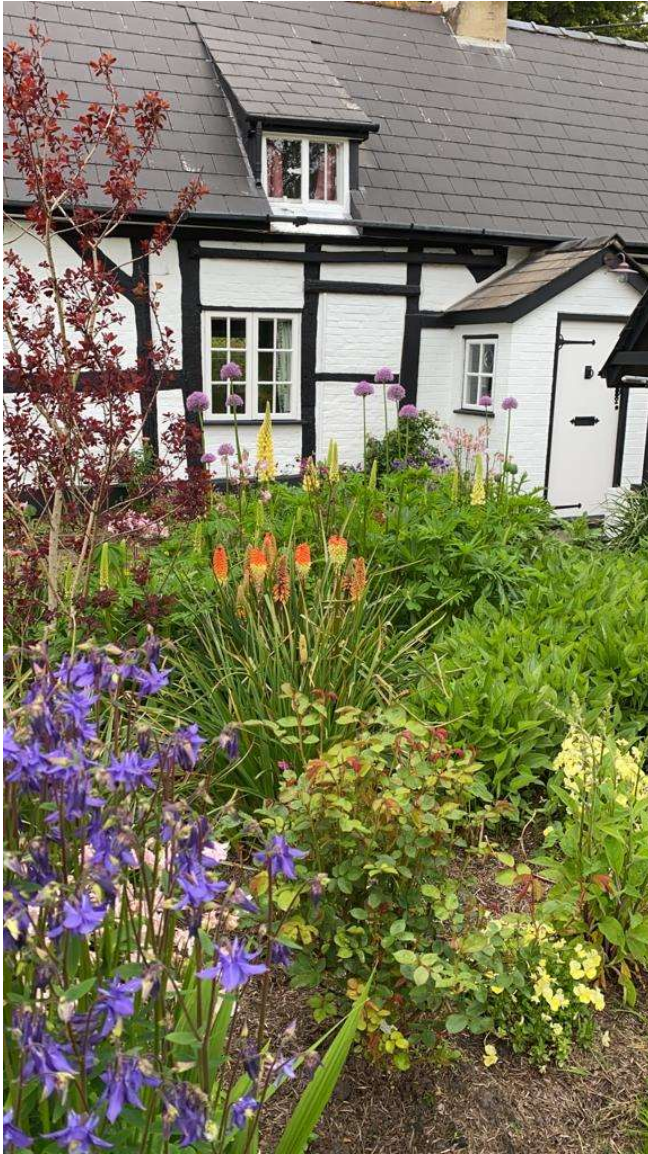
The Front Porch after Works
