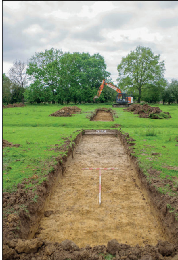
Figure 9: Trench 39, viewed from the northwest
