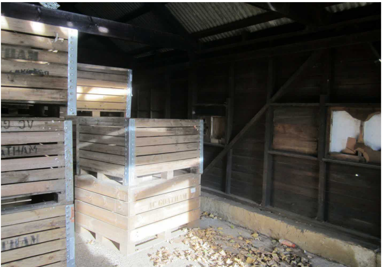
Photo 4. Interior side wall (south-west) and concrete floor of barn.
