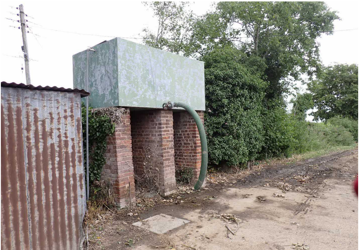
Photo 10. Small water tank
