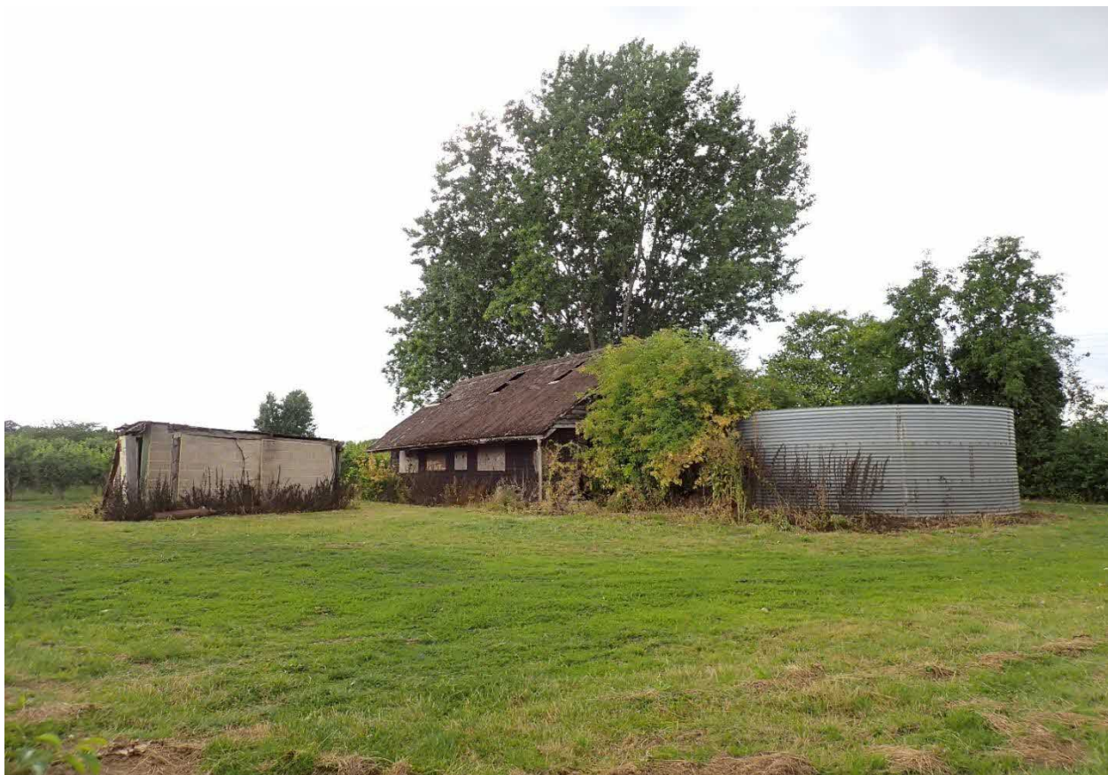
Photo 14. Barn, circular water tank and double garage/store.
