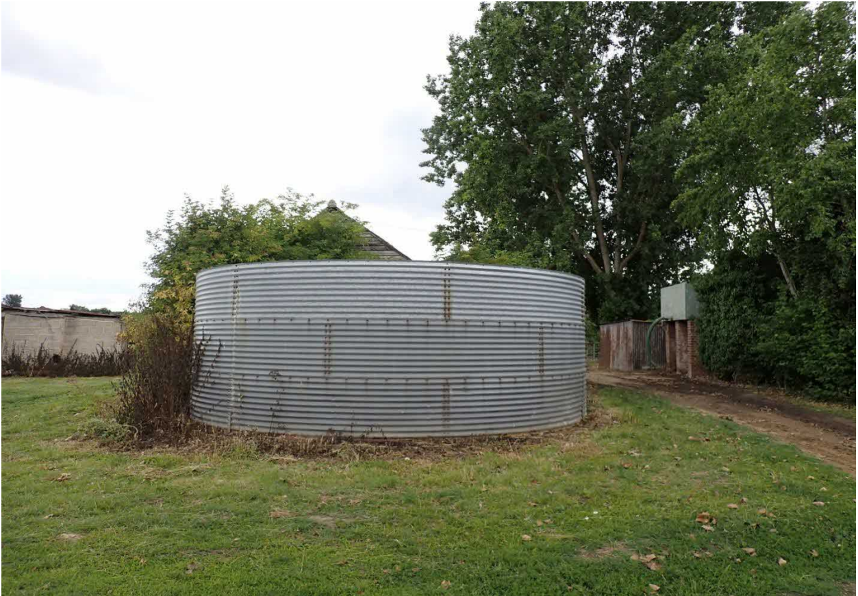
Photo 8. Circular water tank.
