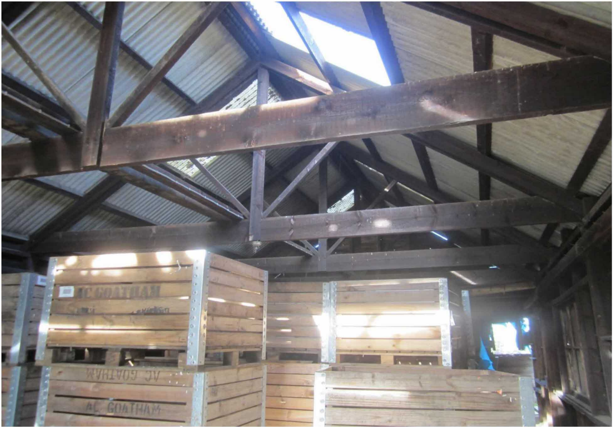
Photo 5. Interior of barn.
