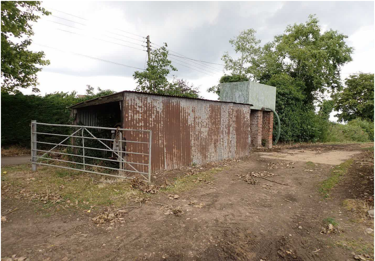
Photo 11. Machinery storage shed with small water tank beyond.
