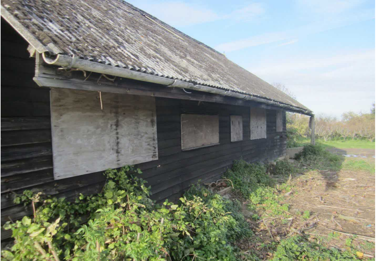
Photo 2. Side elevation of barn.
