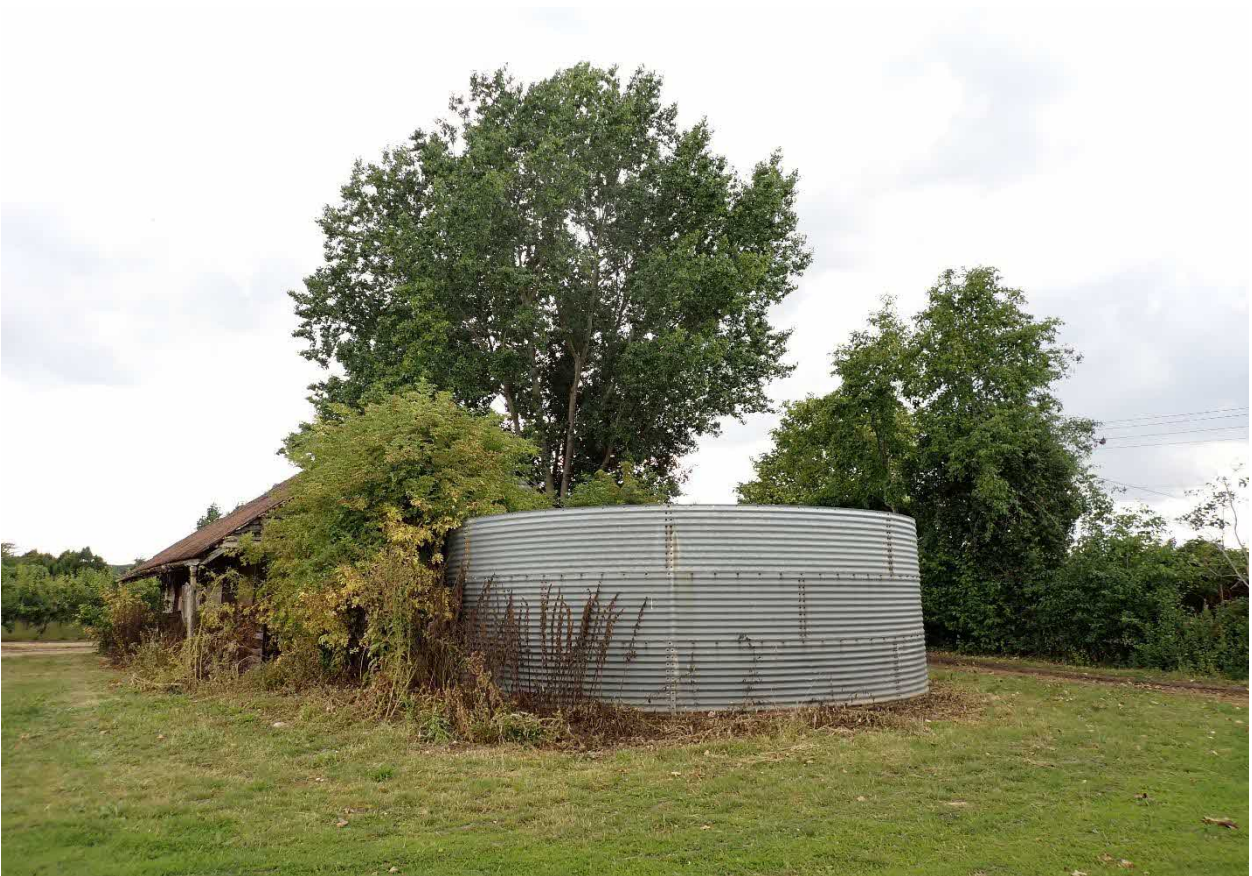
Photo 9. Circular water tank.
