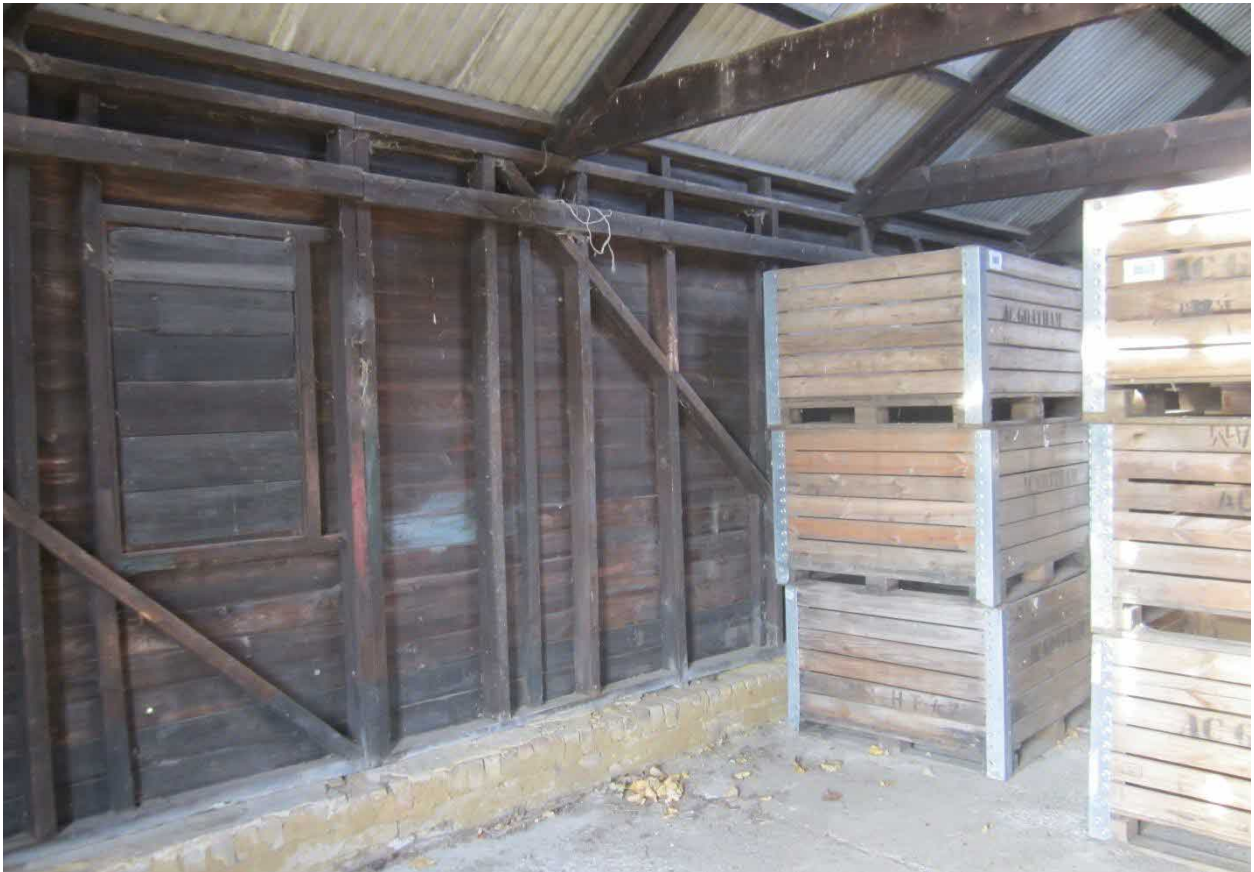
Photo 3. Interior side wall (north-west) and concrete floor of barn.
