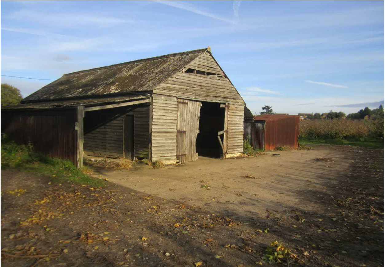
Photo 1. Front elevation of barn and area of hardstanding.
