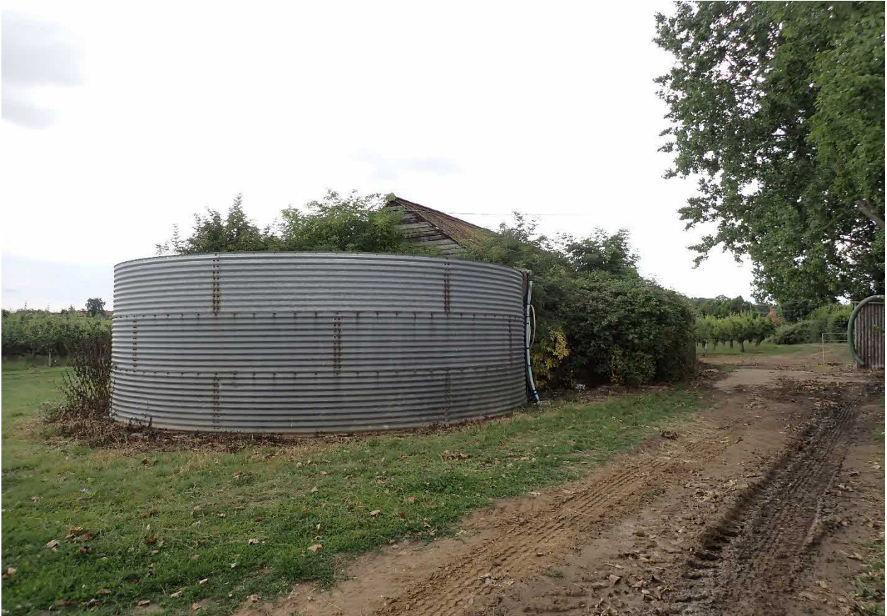
Photo 7. Circular water tank.
