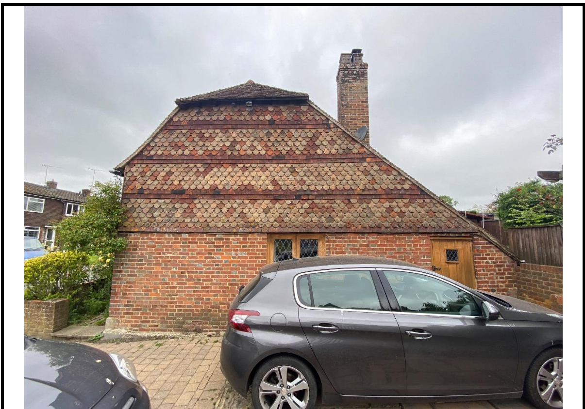
PHOTO 2 – Side (Eastern) Elevation including side door to be replaced.
