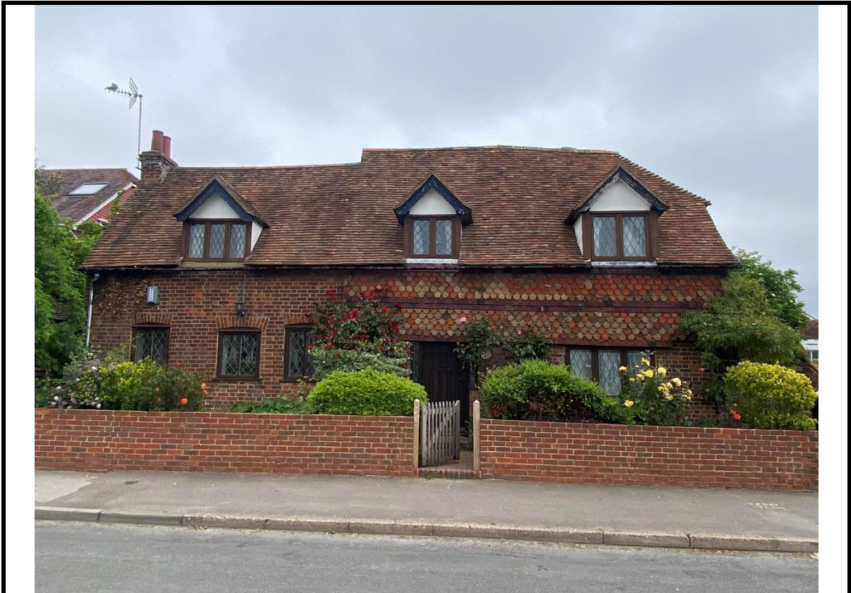
PHOTO 1 – Principal (South) Elevation including 7no. windows and front door to be replaced.
