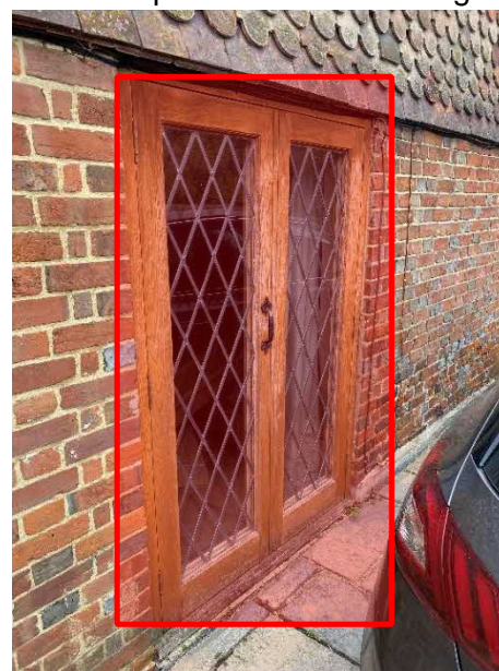
Figure 5: Side door to be replaced.
