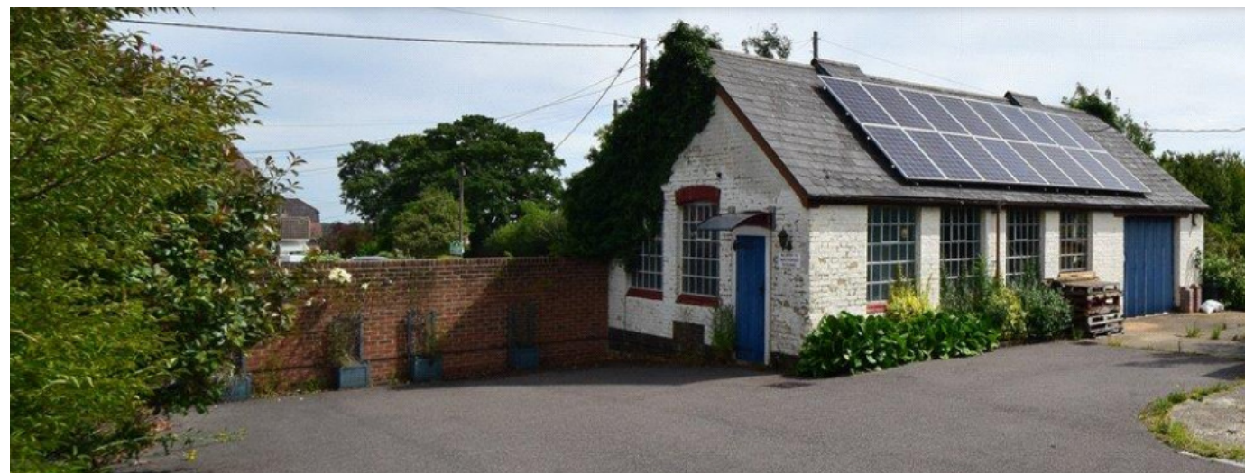
The Old Storage Unit
