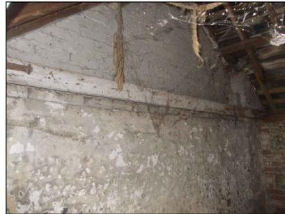
B - Internal view looking north showing brick and flint dividing wall; note tie beam
