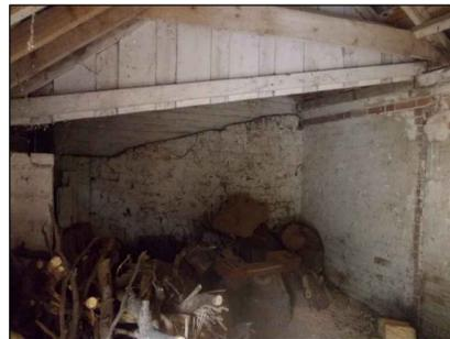
C - Internal view looking north showing composite brick external wall with area of random headers
