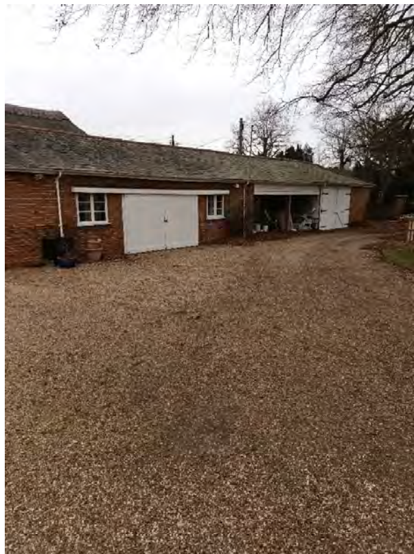
Photo 2: Outbuilding located along northern boundary of the site.
