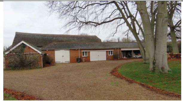
Northern outbuilding, southern elevation.
