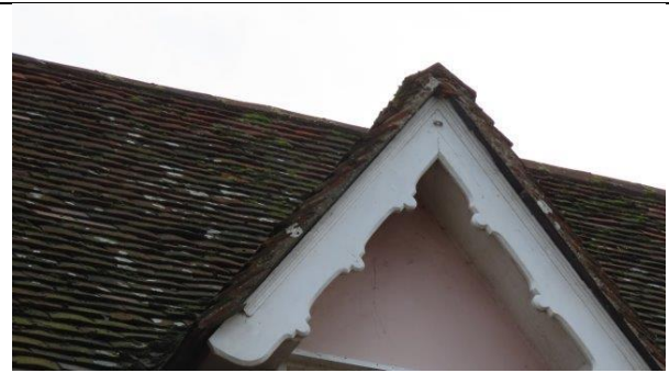
Church Close House, northern elevation dormer gables
