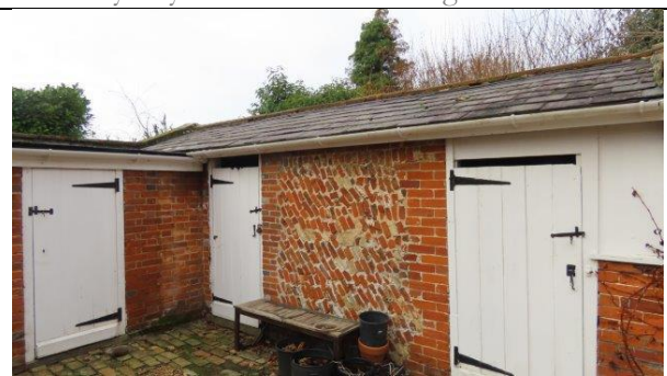
Western outbuilding, eastern elevation
