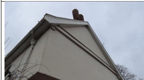
Eastern elevation of Church Close House
