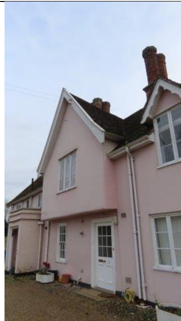
Church Close House, northern elevation
