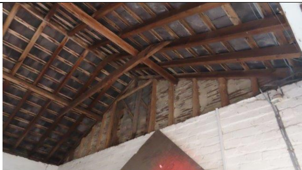
2e Roof space interior of northernmost room in western section.
