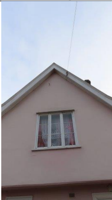
Church Close House, northern elevation
