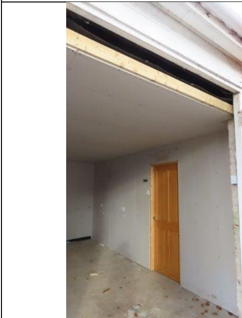
Northern outbuilding interior.
