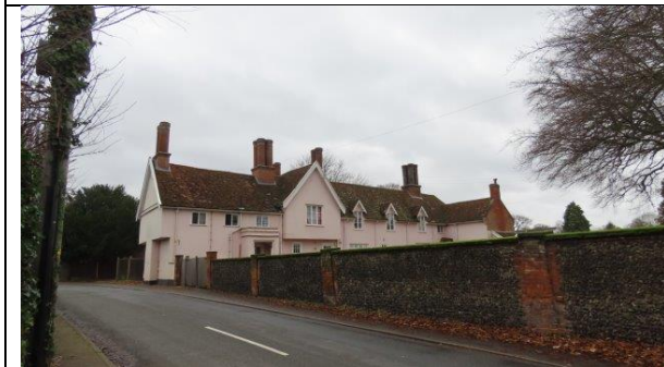
Church Close House from Church Lane, showing north and east elevations.
