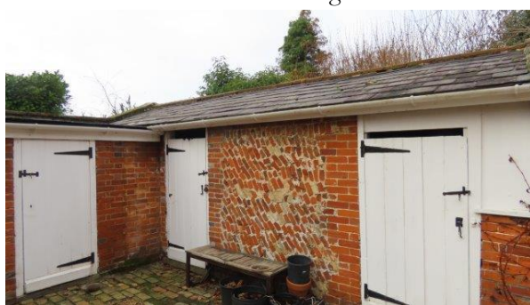
3b Western outbuilding exterior
