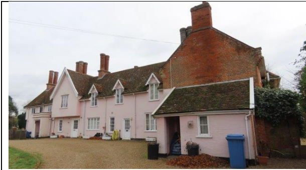
Church Close House, northern elevation
