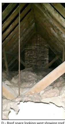
D - Roof space looking west showing roof structure (purlins/struts/metal ties) indicative of the 19th c. Brick chimney likely 17 c (lower section)
