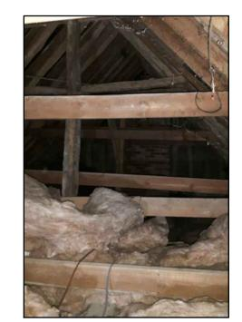
G - Roof space looking north east showing mutilated crown post roof structure to likely
