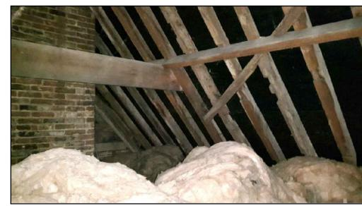
F - Roof space looking east showing likely 17 c chimney stack and roof structure (purlins, ties) of mainly reused timber sections
