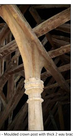
B - Moulded crown post with thick 2 way bracing in crosswing
