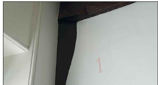
E - Principal jowelled post with tie beam and chamfer stop (end wall of original crosswing)
