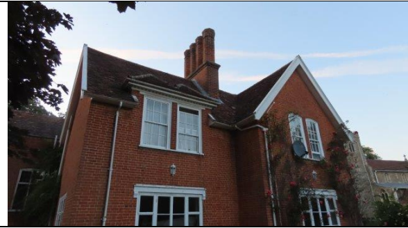
Photo ref 8. Southern elevation of southern extension
