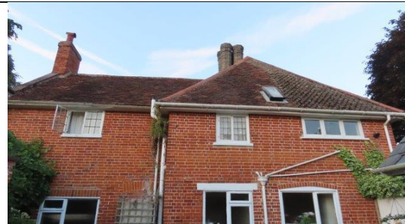
Photo ref 10. View of house from courtyard, showing western elevations.
