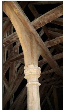
B - Moulded crown post with thick 2 way bracing in crossing
