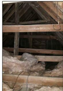
G - Roof space looking north east showing mutilated crown post roof structure to likely original Hall and much later structural alterations
