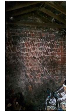
I - Internal view looking west showing composite brick external wall with area of random headers
