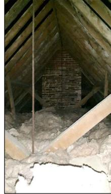
D - Roof space looking west showing roof structure (purlins/struts/metal ties) indicative of the 19th c. Brick chimney likely 17 c (lower section)
