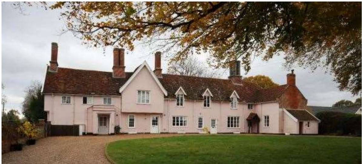
Figure 2 – View of the main house looking south.
