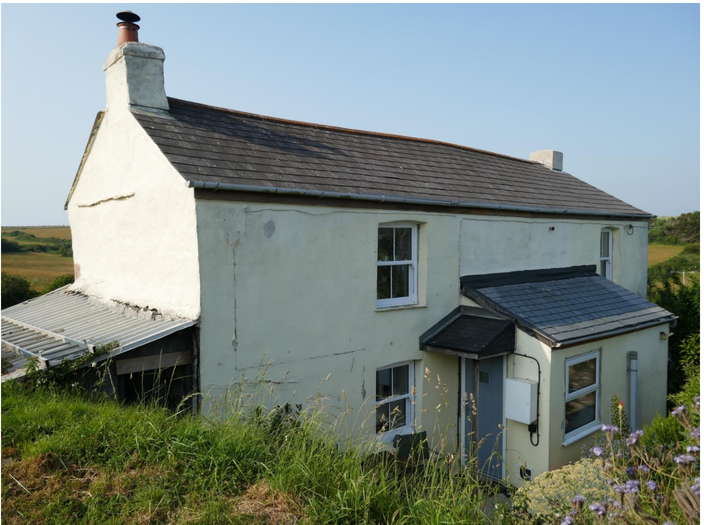
Figure 1. Southern and western aspect of the building.
