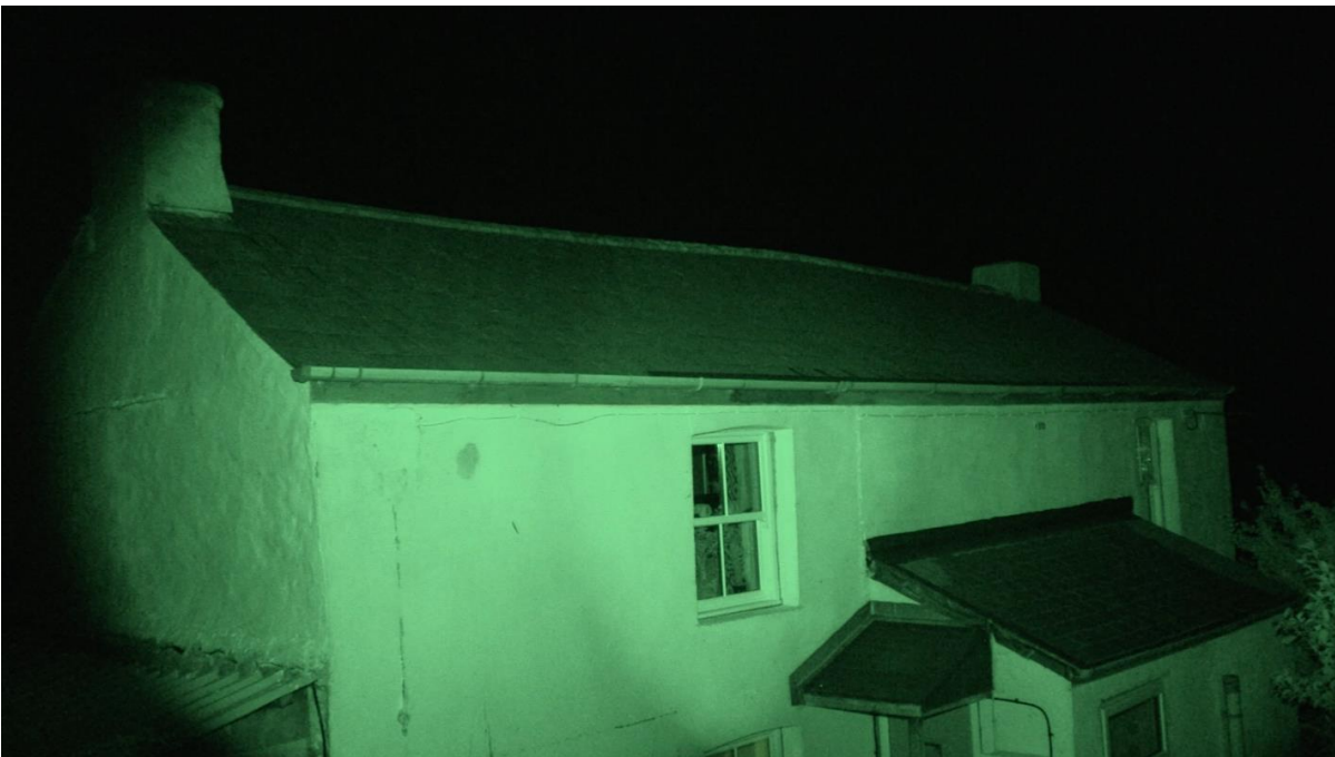
Figure 7. Infrared illumination for surveyor 1 on 11 August 2023.
