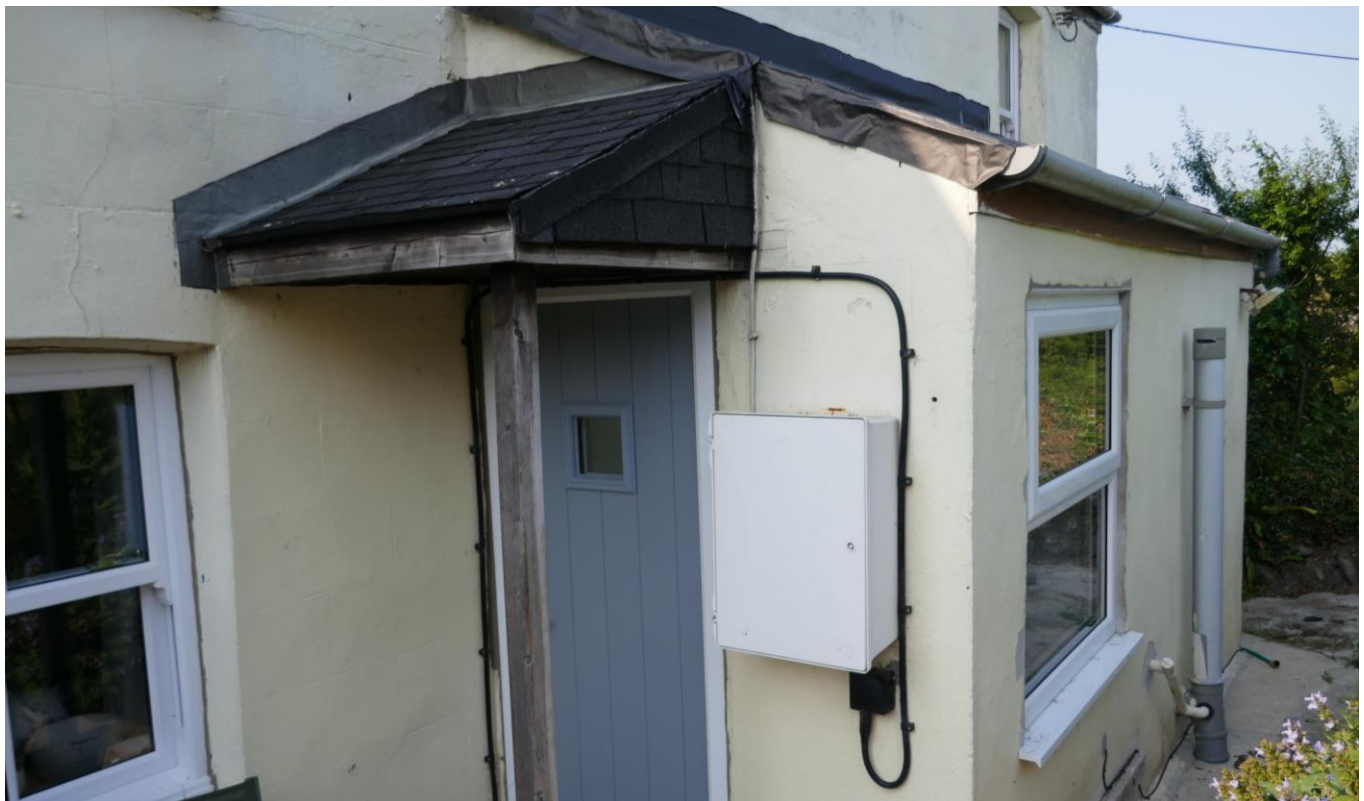
Figure 5. Porched entrance on southern aspect.
