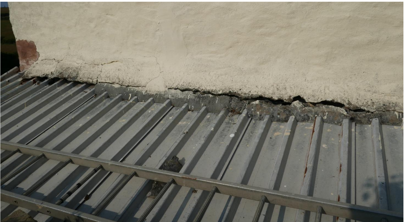
Figure 3. Large gaps at the junction of the house and the lean-to on the western aspect.
