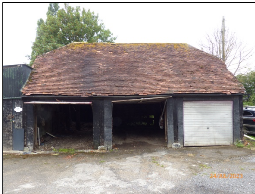
Figure 1: Southern elevation of garage.
