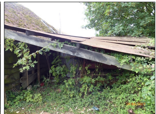
Figure 4: Metal clad extension on northern elevation.
