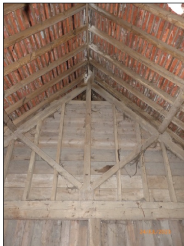
Figure 5: Interior view of eastern part of the building, showing timber partition wall.
