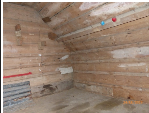
Figure 6: First floor section with wooden panelling beneath clay tiles and behind side panels.
