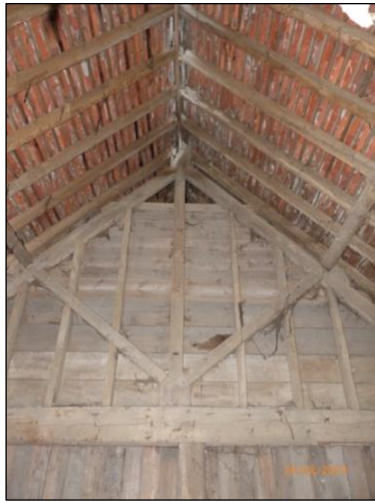
Figure 5: Interior view of eastern part of the building, showing timber partition wall.
