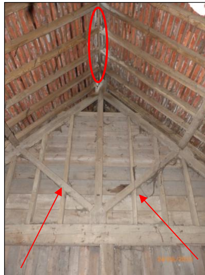
Figure 7: Interior view of garage showing potentially suitable roosting locations.
