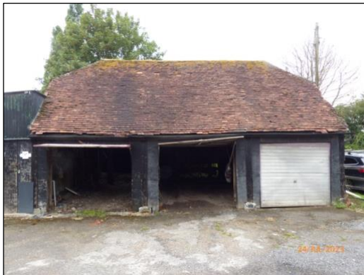
Figure 1: Southern elevation of garage.
