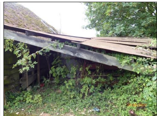
Figure 4: Metal clad extension on northern elevation.
