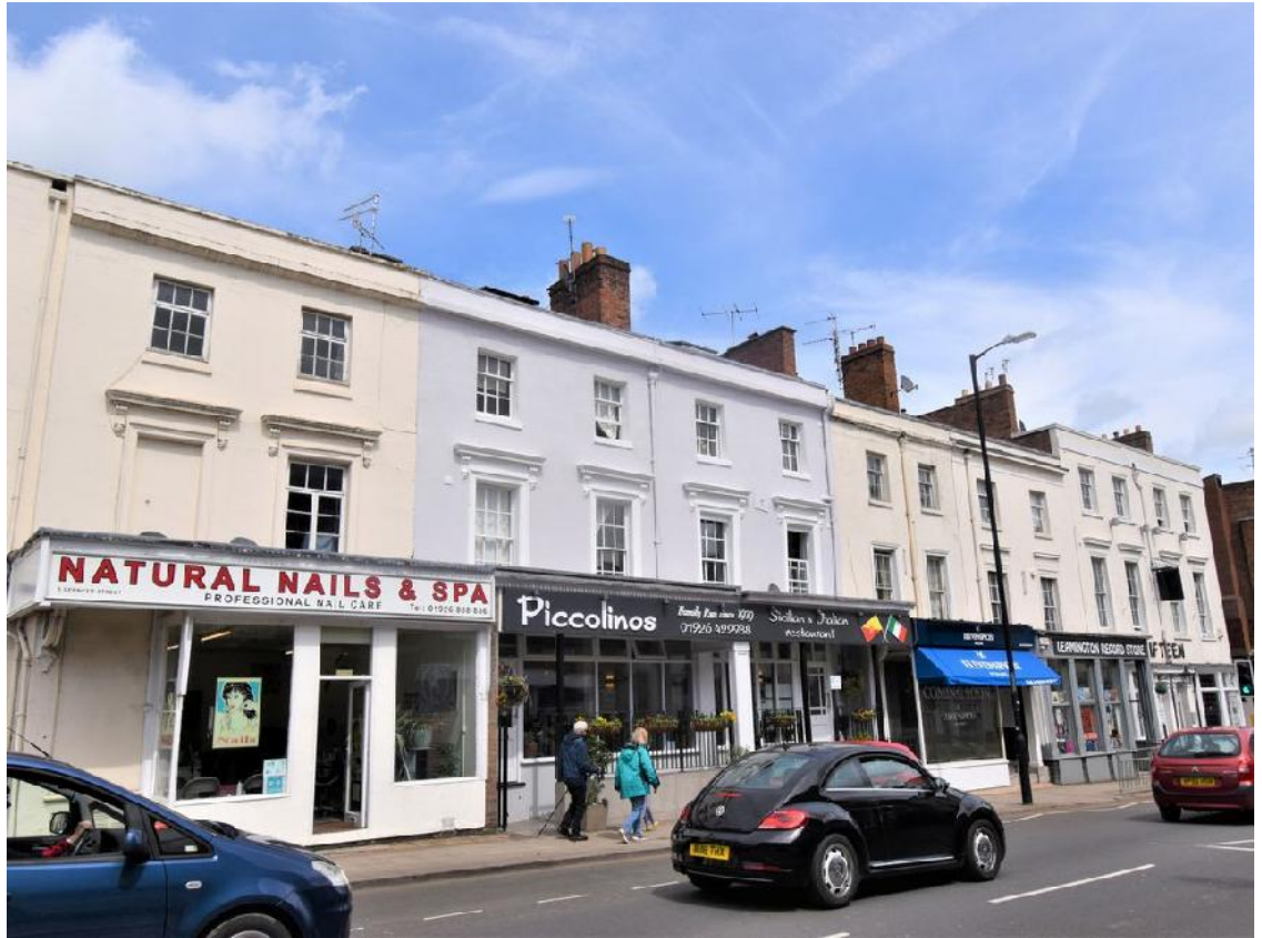
Figure 2 – Street frontage, showing nos. 5 – 13 Spencer Street, Leamington Spa
