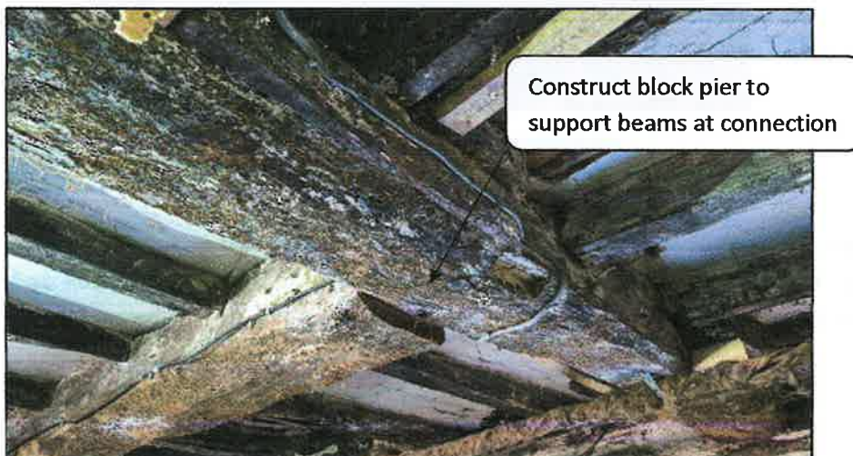
Photograph 4: Existing timber floor beam connection
