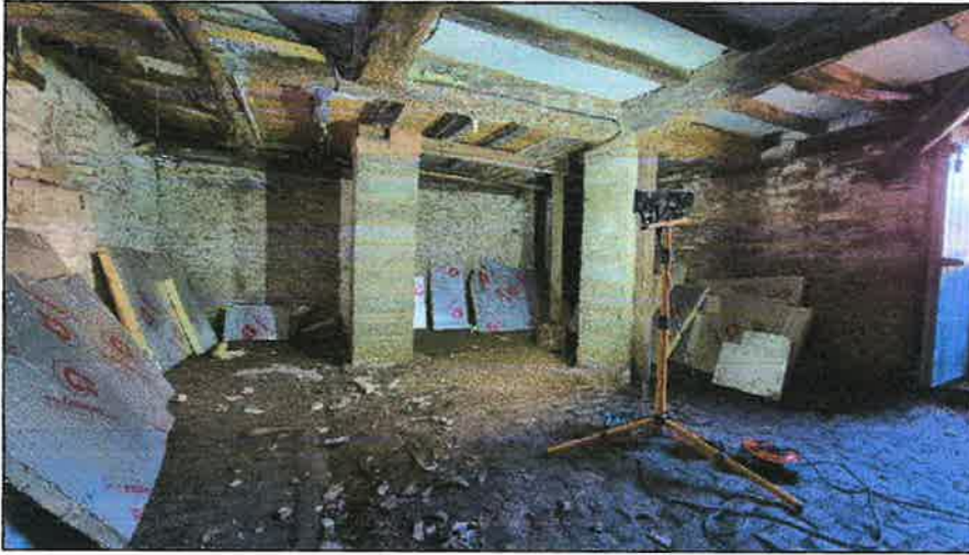
Photograph 1: View of Cellar looking towards the rear of the property
