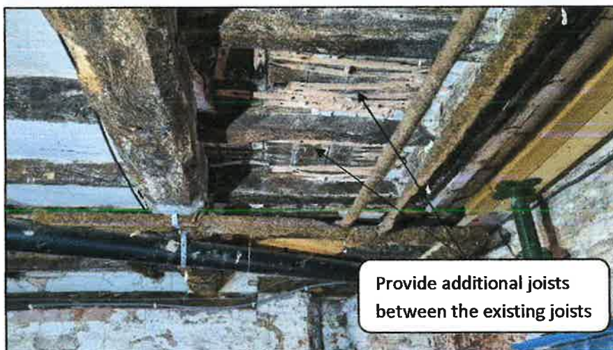
Photograph 6: Floor adjacent to hearth
