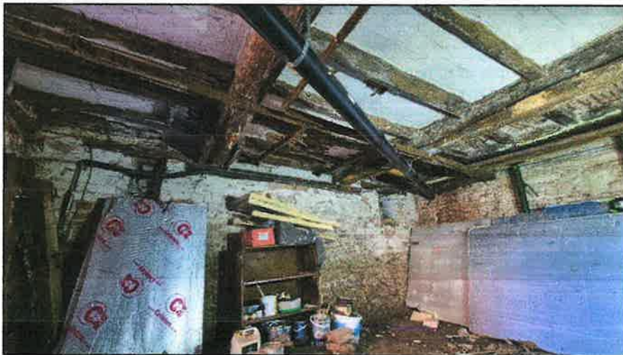
Photograph 2: View of Cellar looking towards the front of the property
