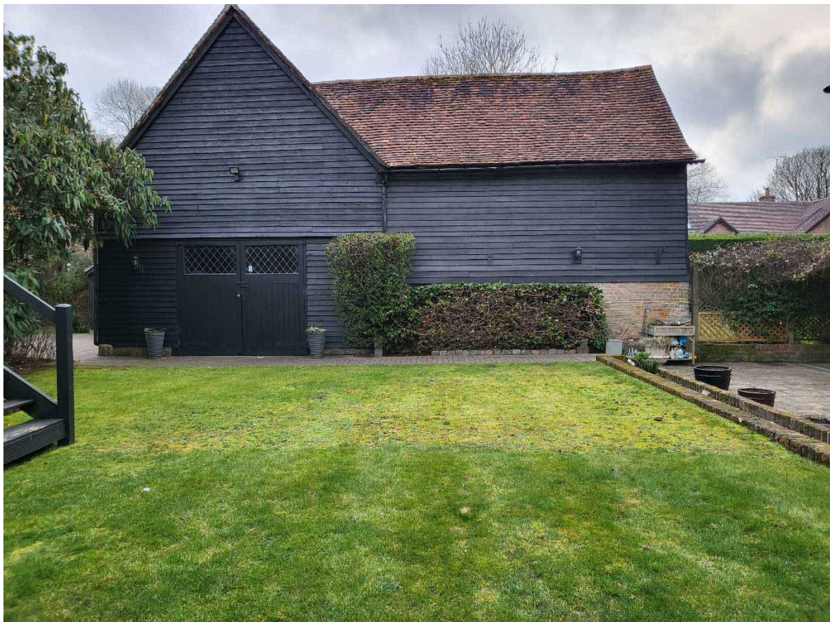
Figure 3. The Barn now in use as a garage viewed from the North.
