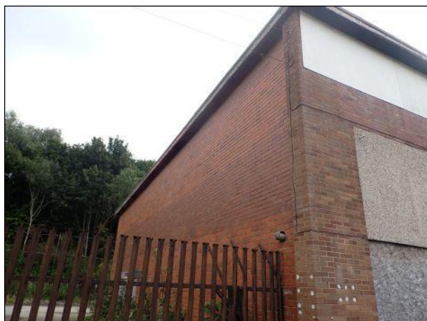
Photo 5: Building 1, northern elevation (the former workshop)
