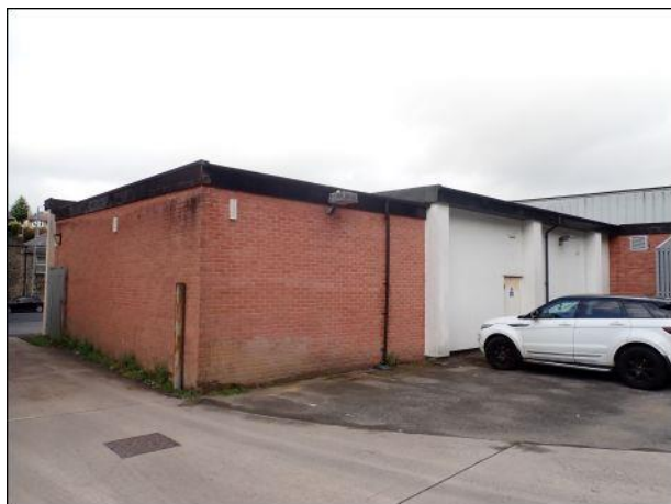
Photo 9: Building 1, eastern elevation, southern end (SPAR retail outlet)
