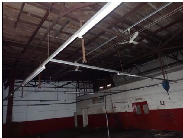
Photo 12: Building 1, internal area (northern end, former workshop)
