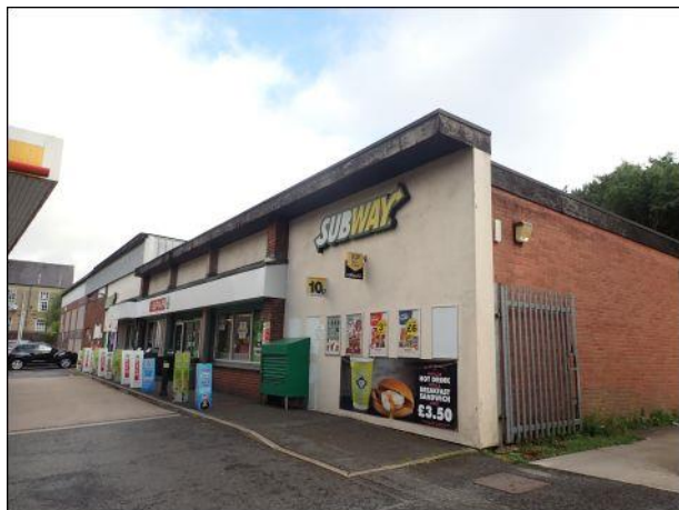
Photo 7: Building 1, western elevation, southern end (SPAR retail outlet)
