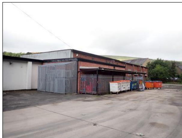
Photo 10: Building 1, eastern elevation, central section (SPAR retail outlet)
