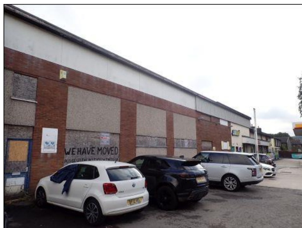
Photo 6: Building 1, western elevation, northern end (the former workshop)
