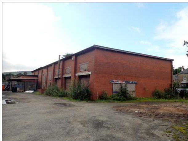
Photo 11: Building 1, eastern elevation, northern end and northern elevation (former workshop)
