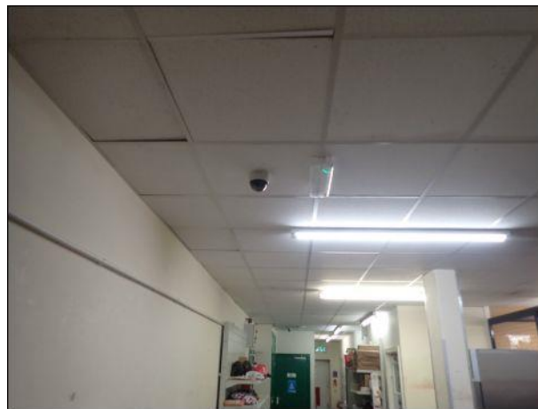
Photo 16: Interior of Building 1, southern end (occupied SPAR retail outlet)
