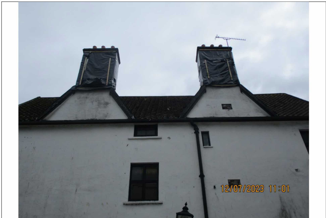
PHOTOGRAPH 2 – View from Queen Charlotte Street (high level part of elevation)
