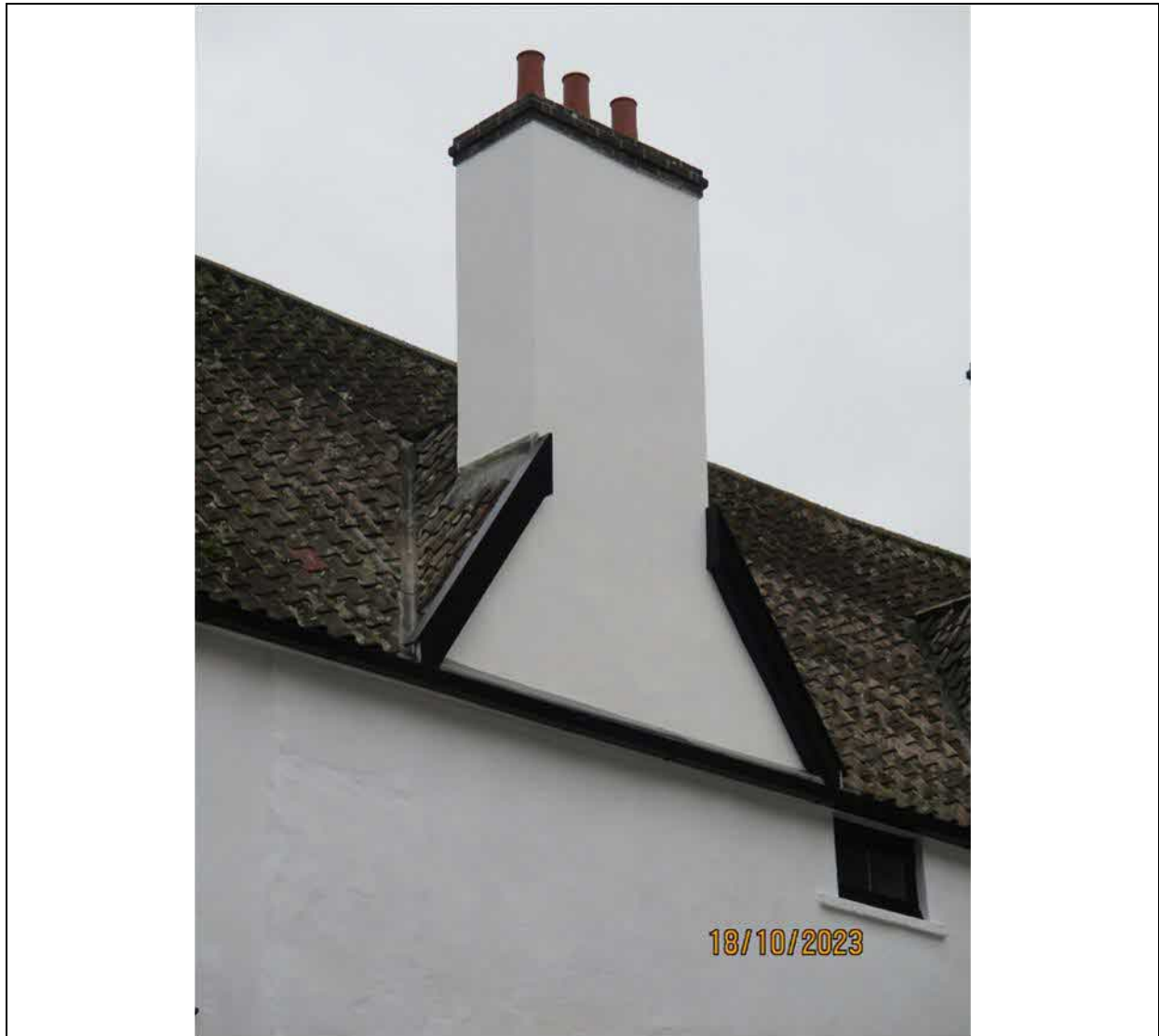
PHOTOGRAPH 5 – View of North Gable Chimney Stack
