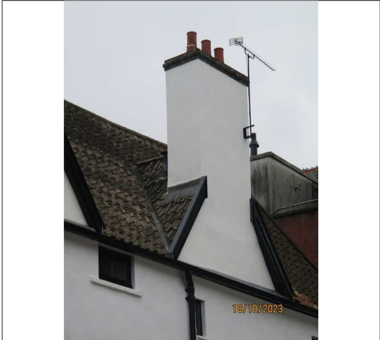
PHOTOGRAPH 4 – View of South Gable Chimney Stack
