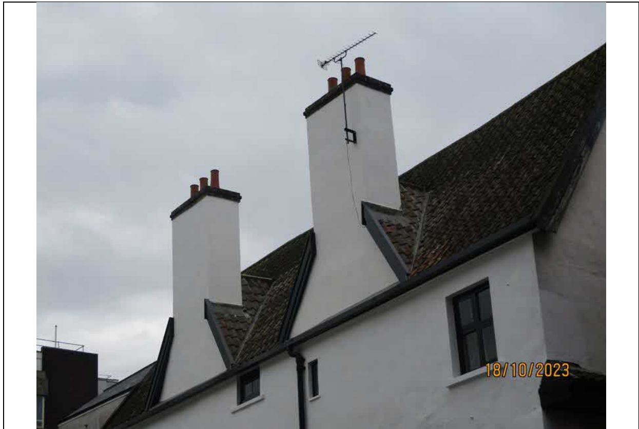
PHOTOGRAPH 3 – View from Queen Charlotte Street (high level part of elevation)
