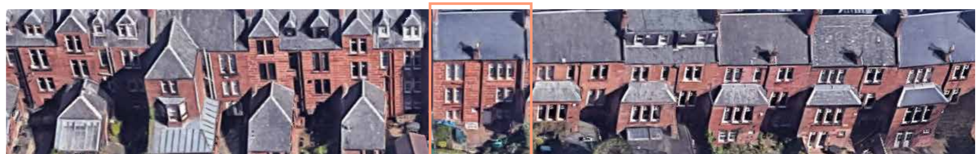
^ Fig 6.1 27 Kingsborough Gardens presents the only instance where the FF and GF windows do not line through with on another.
