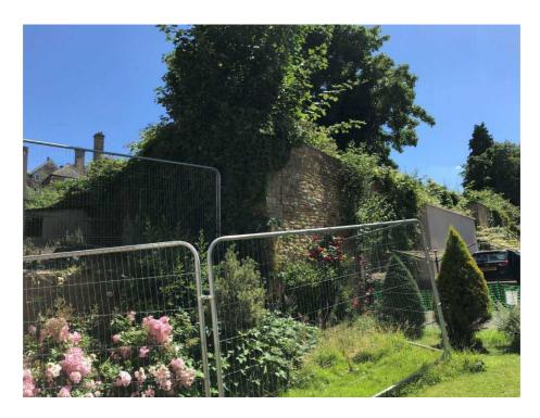
View of the failing retaining wall from the front of the residential flats. Note required security fencing in place and the obvious fracture lines in the retaining wall.
