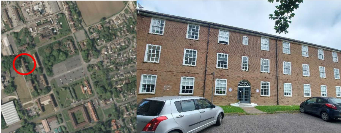
Figure 1: Aerial view of the site Figure 2: Bowen House
