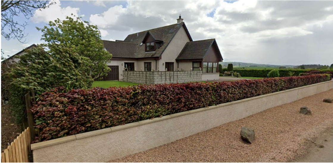
View of the house from the North
