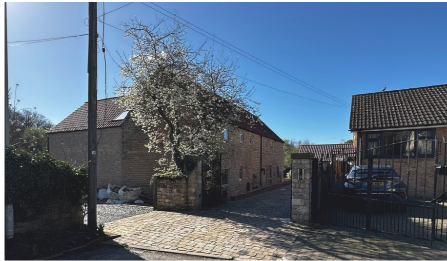
Top Image: View from garden towards rear of property Bottom Image: View from corner of Low Street towards front of property
