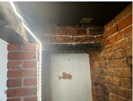
Please see photos below of a recent, non-listed inglenook repointing undertaken showing original condition, raking out of mortar, and finished condition. Raking out of mortar is carried out by hand using a range of tools depending on the condition of the bricks – great care is taken to prevent damage.
