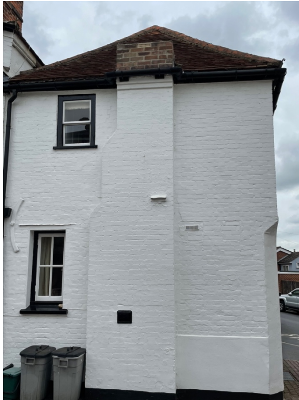
West Elevation showing former chimney stack previously reduced.
