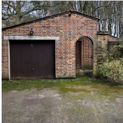
Photo 6 , Photograph looking towards garage 1.
