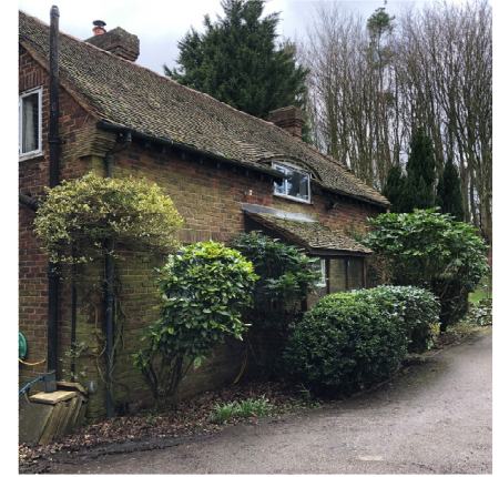
Photo 4 , Photograph looking towards the front of the property.
