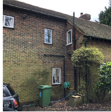
Photo 3 , Photograph looking towards the front of the property.
