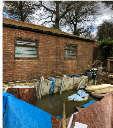
Photo 7 , Photograph looking towards garage 1.
