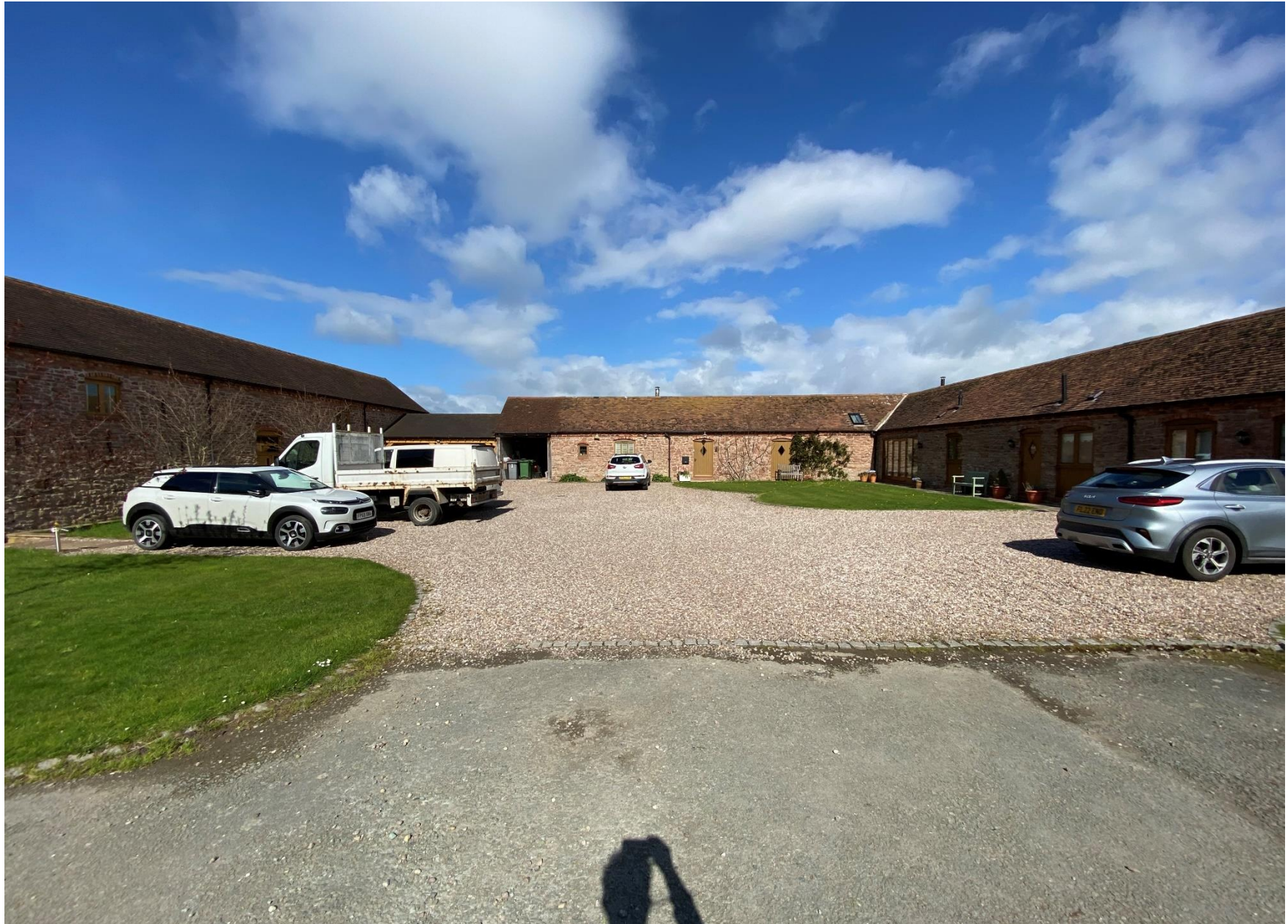
Figure 17 – The overall Heath Farmstead site. The historic layout is retained, despite the site having been converted to residential.
