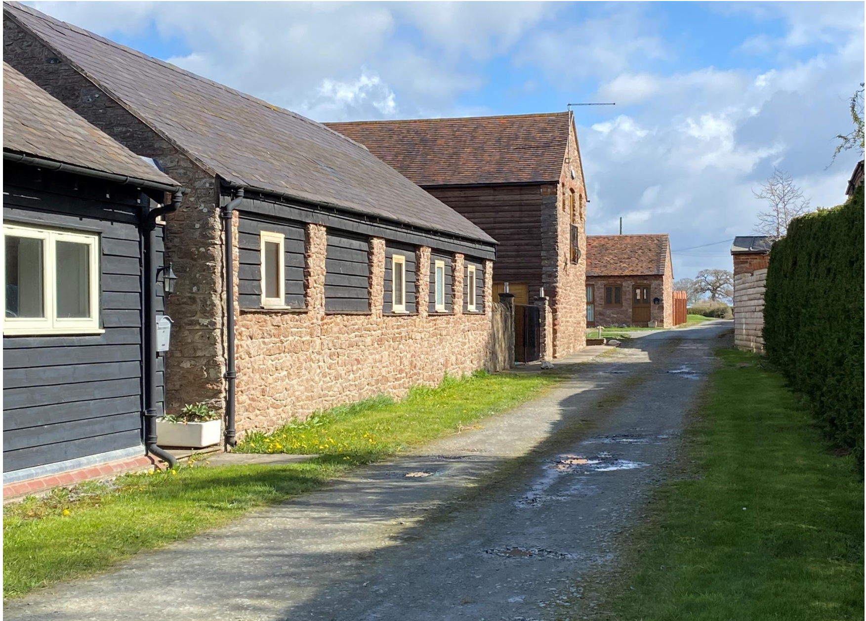
Figure 18 – Further evidence of the Heath Farm’s conversion, including the replacement of windows.
