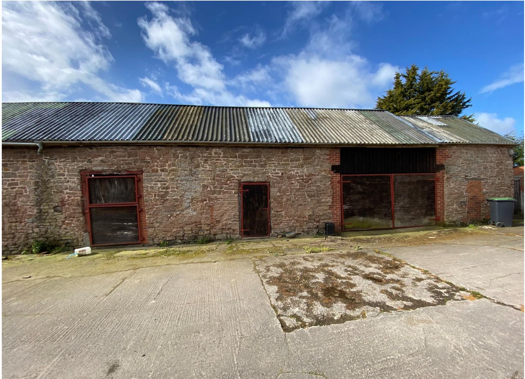
Figure 12 – Threshing Barn converted to Cowhouse at Far Broadway Farm site.
