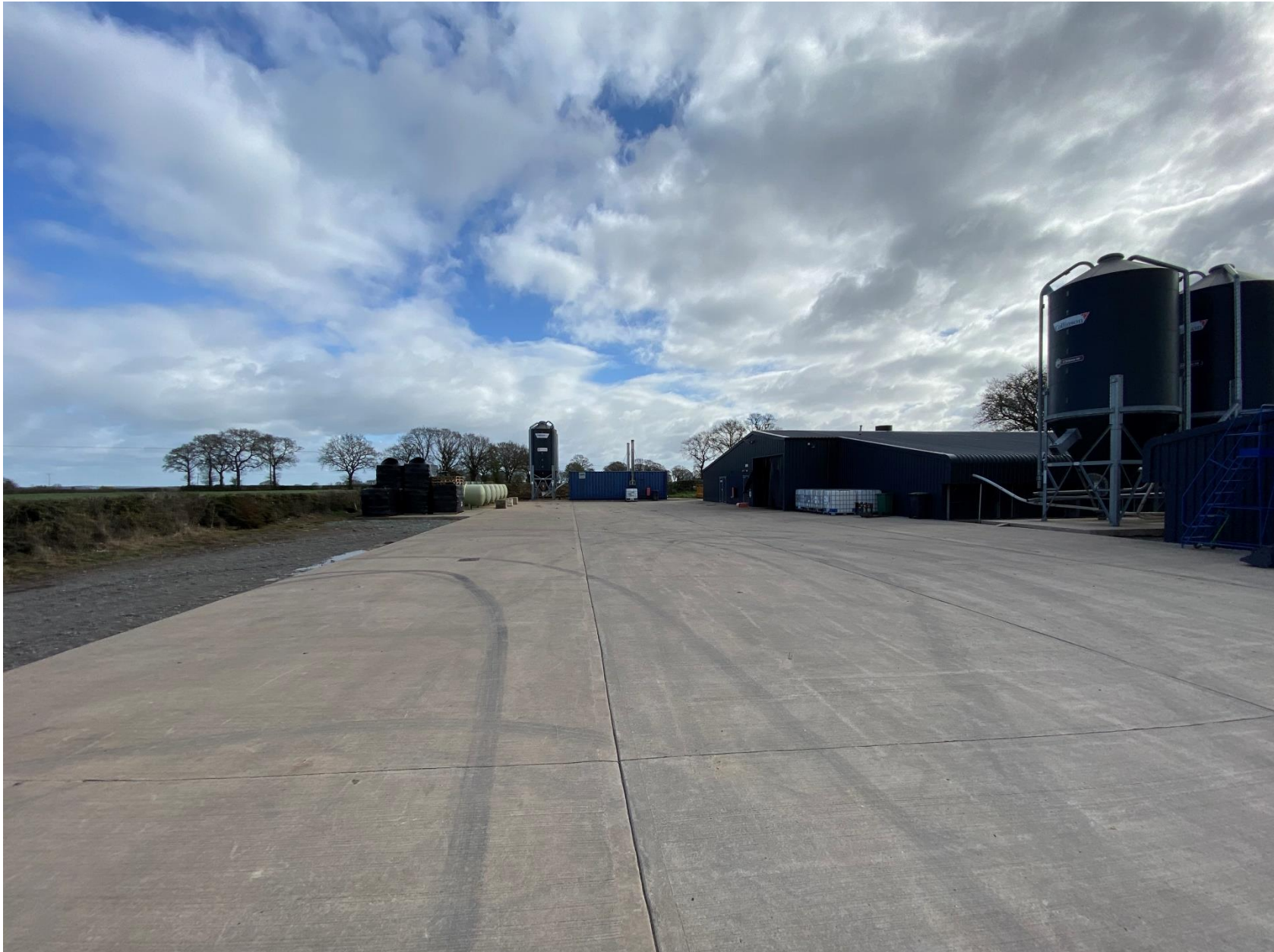
Figure 7 – The farm already contains within it 4 poultry sheds with associated infrastructure.
