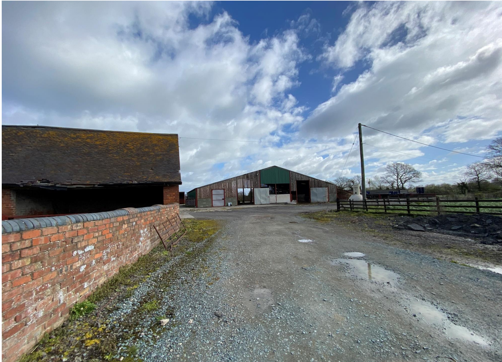
Figure 14 – Further modern agricultural buildings within the Far Broadway Farm site.
