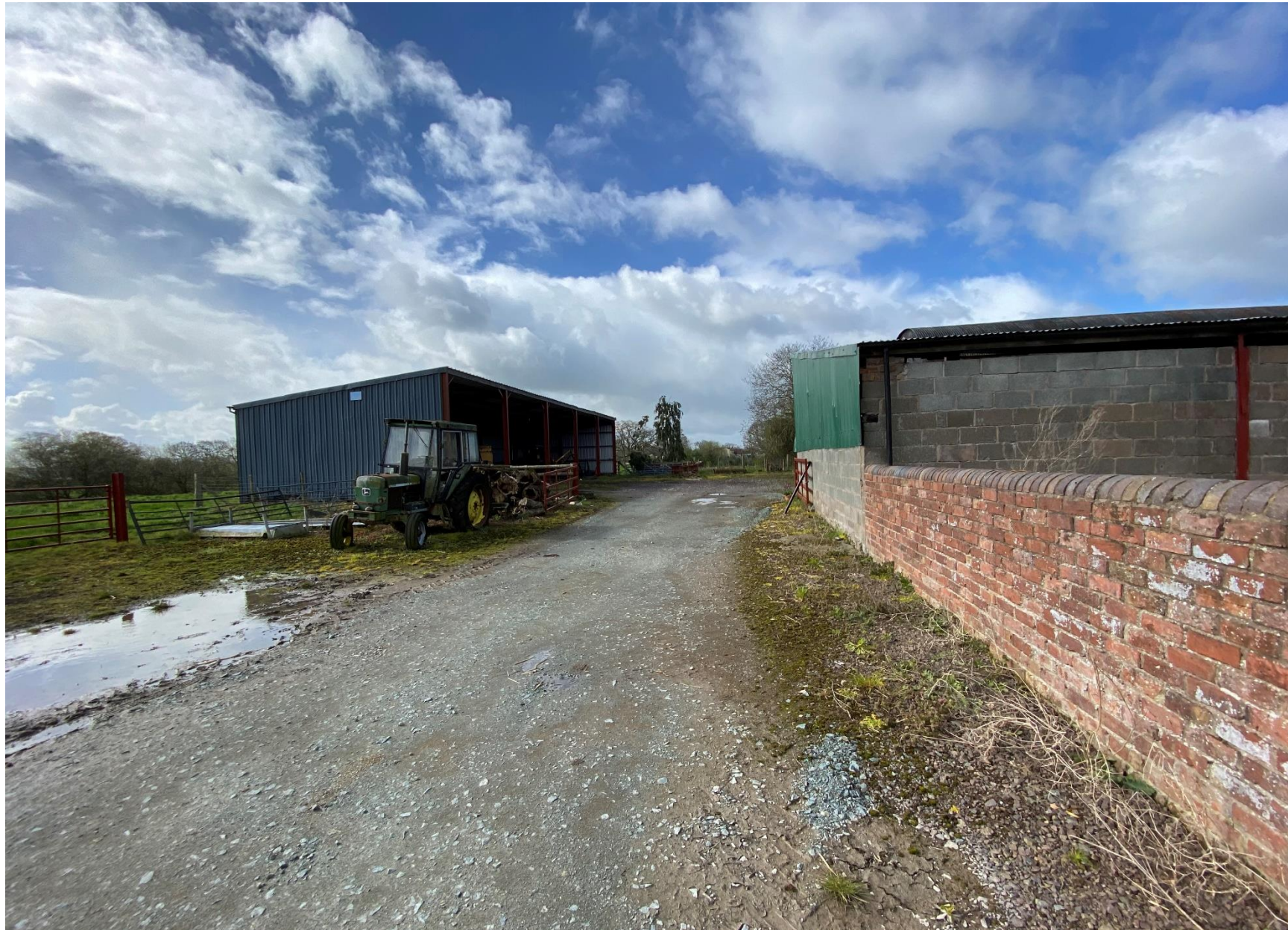
Figure 13 – There has been the erection of further modern agricultural buildings within the setting of Far Broadway Farm which has already impacted the setting of the heritage assets found here.
