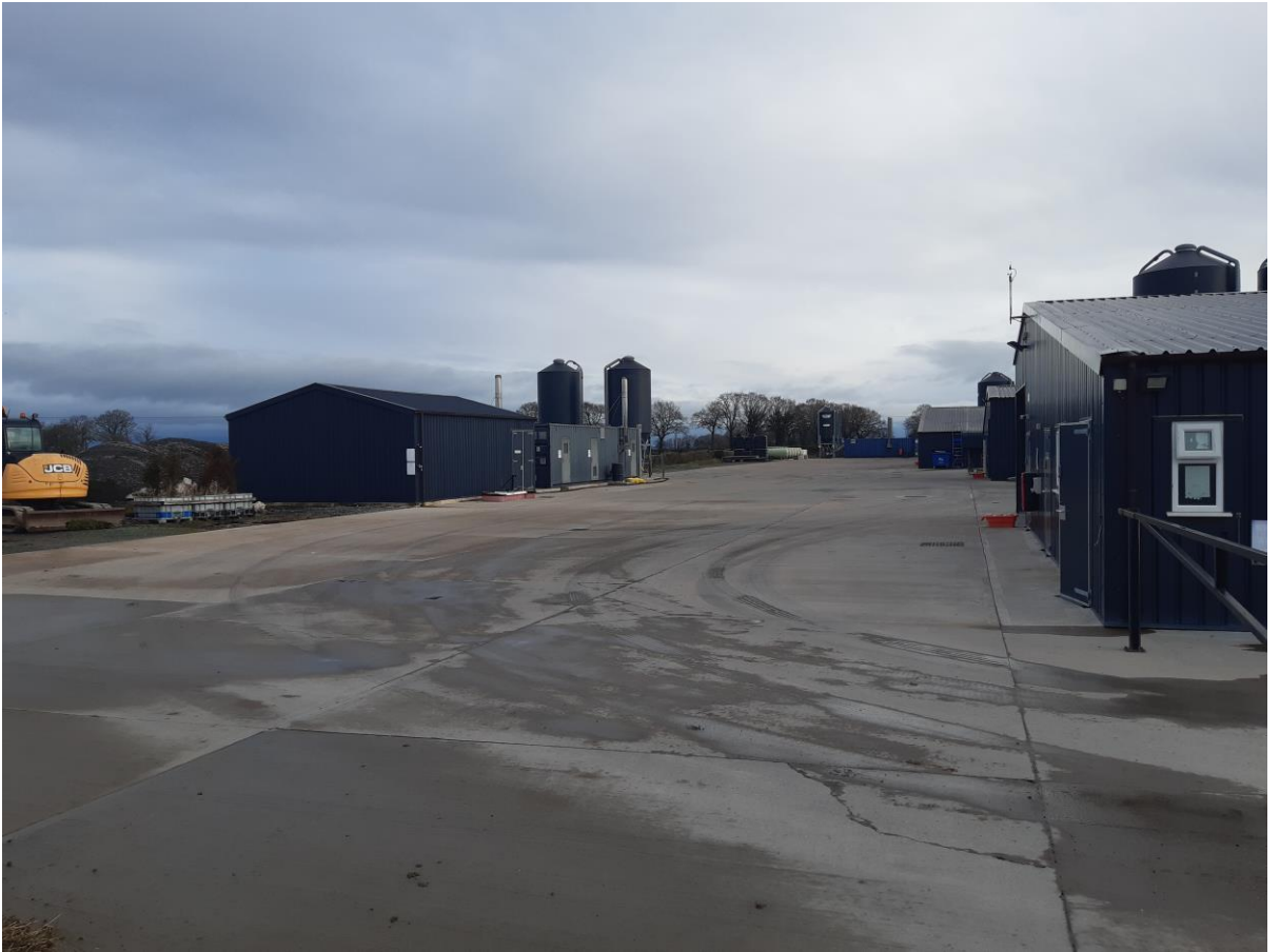
Figure 6: Existing complex of poultry shed to the south
