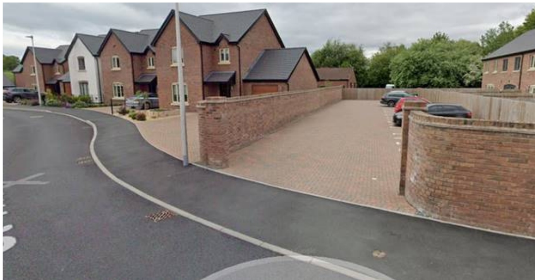
Photo 3 – Access to a parking court with boundary walls immediately adjacent to the rear of the footway of the highway boundary.
