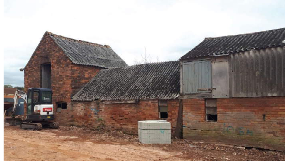
Two storey Cattle Barn and attached Milking Parlour, with the now demolished wing to the right.
