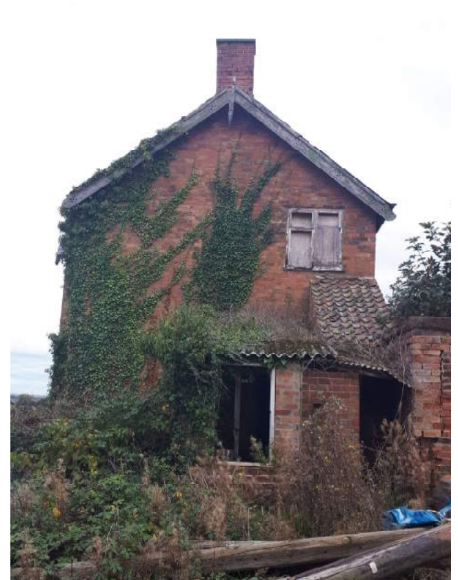
North East elevation with outhouse in the foreground
