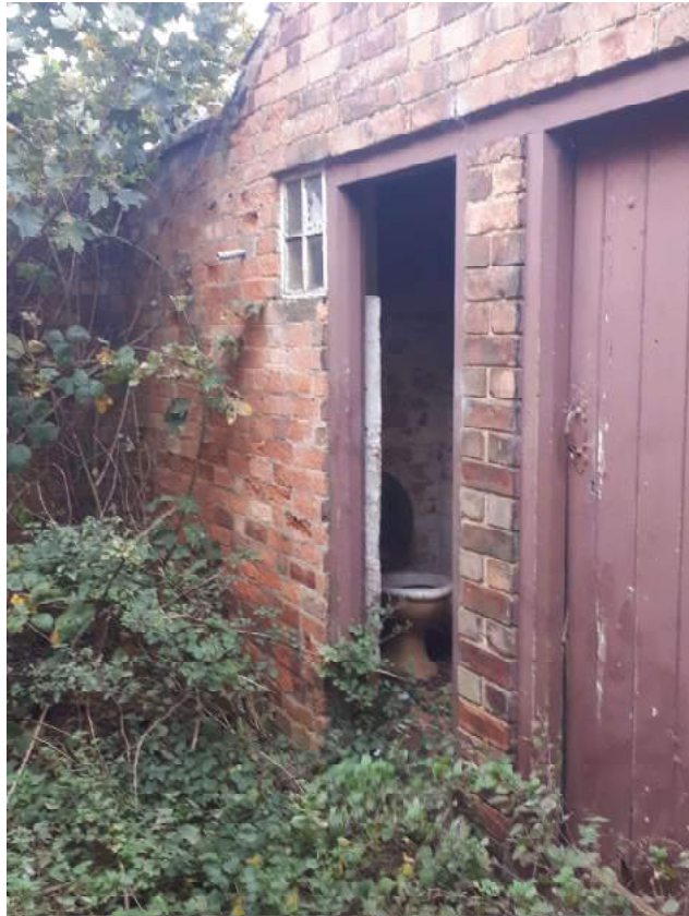
Outhouse believed to have been constructed prior to 1948
