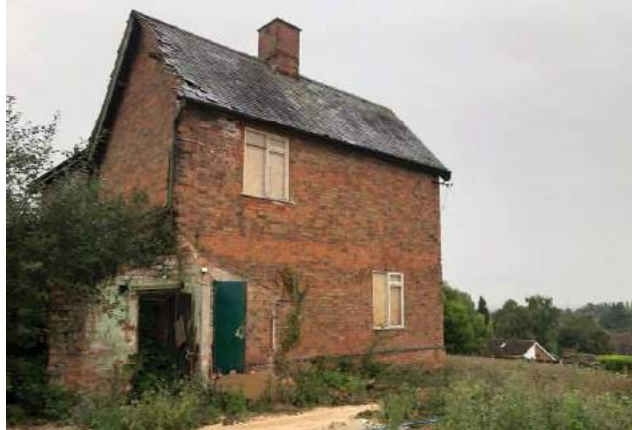
South West elevation of Farmhouse. The line of the partially demolished wing can be seen within the brickwork. To the far left of the picture is the remaining section of the wing which currently houses a WC.
