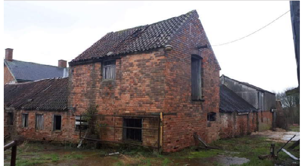
Two storey Cattle Barn, with attached Milking Parlour beyond to the right
