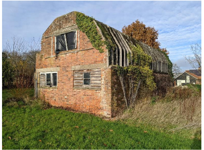
Photo 2 South and east elevations of the existing barn
