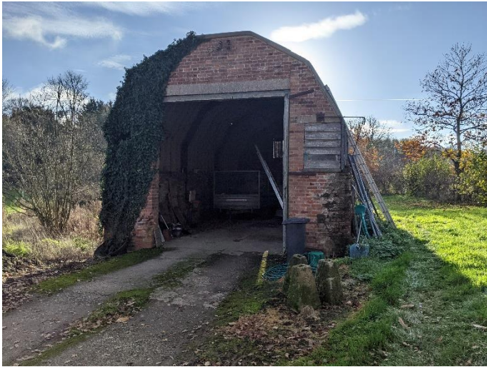
Photo 1 North elevation of existing barn
