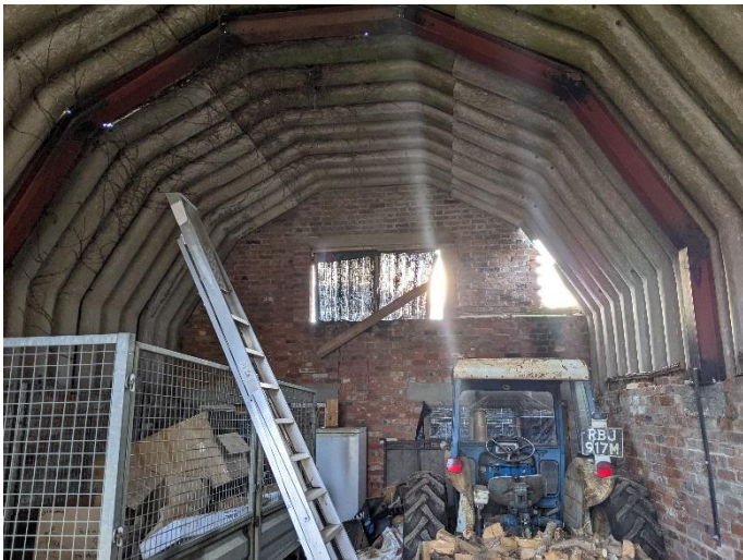
Photo 3 Internal view of existing barn
