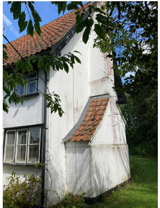
South Elevation from East
