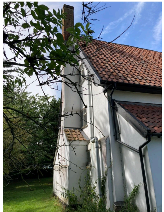
South elevation from West
