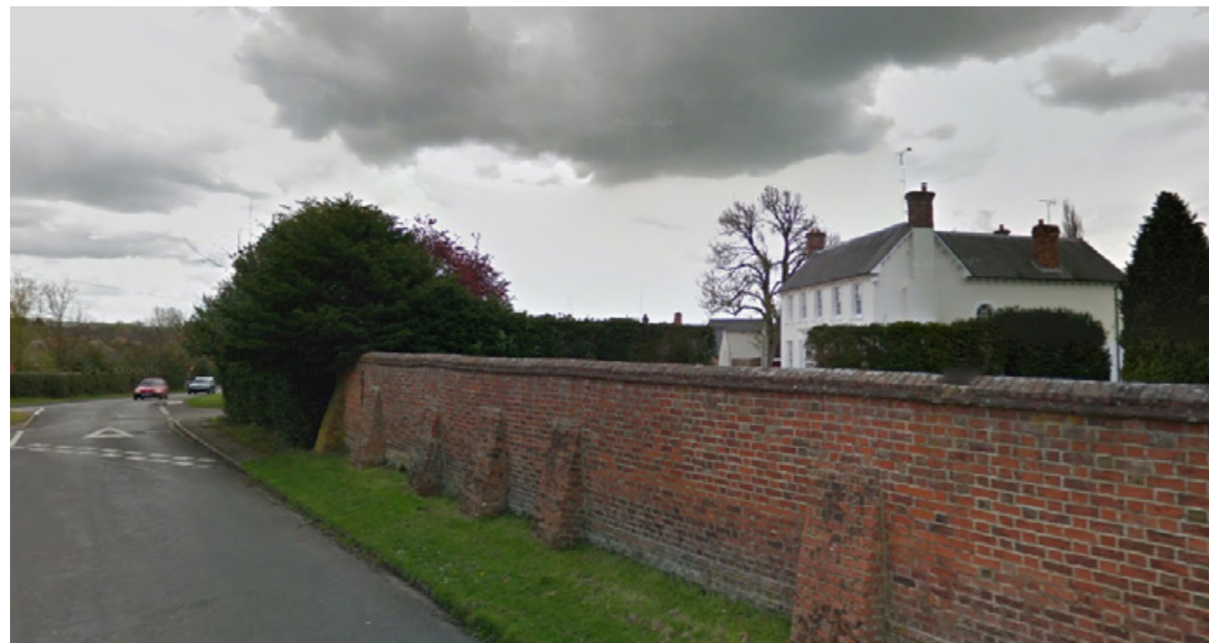
Fig 8. View of the brick buttress wall flanking the front of the site and Side (North) elevation of Stoke Lodge.
