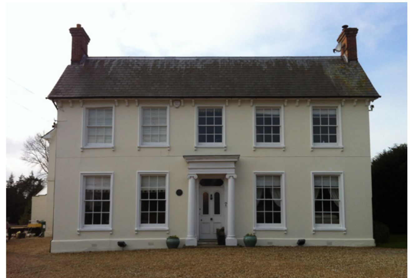
Fig 3. Front (East) elevation view of Stoke Lodge house. EV charging post to be located off south elevation of house (left of picture) out of view of principle front elevation of Stoke Lodge.
