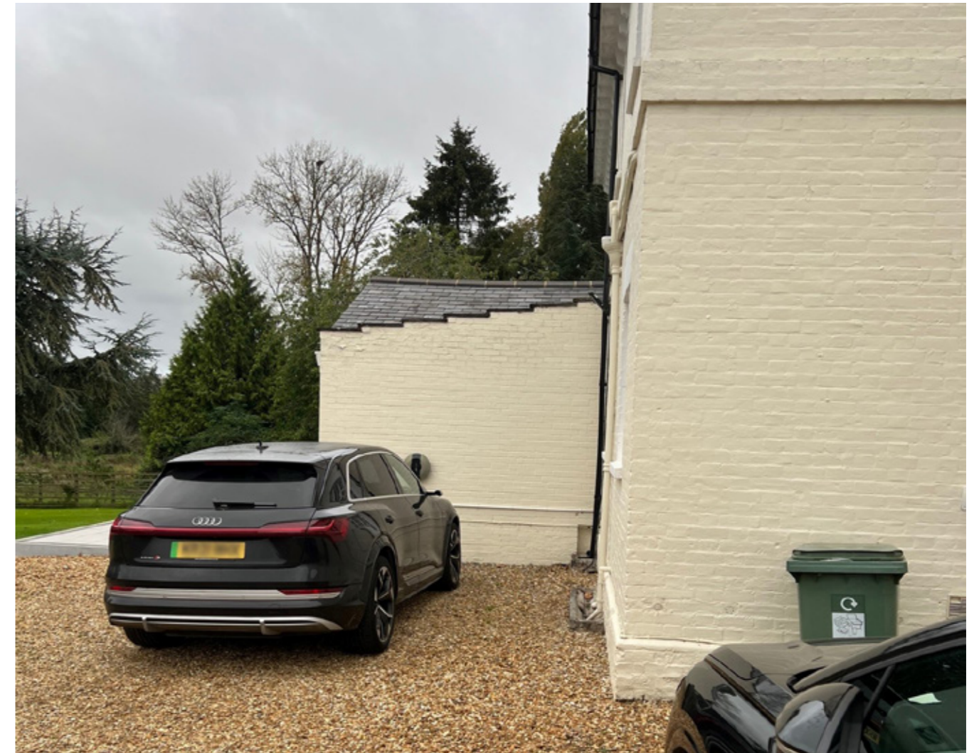
Fig 10. Picture in context showing the existing electric vehicle (EV) charger fixed to the East facing external wall of a rear projecting section of the Stoke Lodge building. The proposal removes the EV charger and conduit from the wall and provide a free-standing post away from the building in the corner to the right of the picture which is out of sight from the principle entrance elevation of Stoke Lodge.
