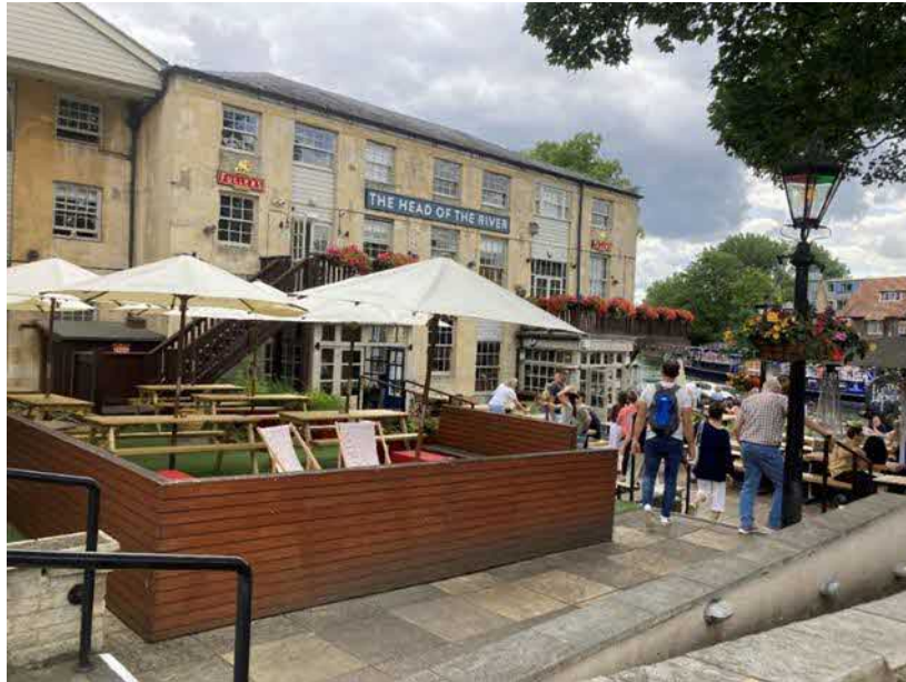
Above – Front of former warehouse and existing beer garden
