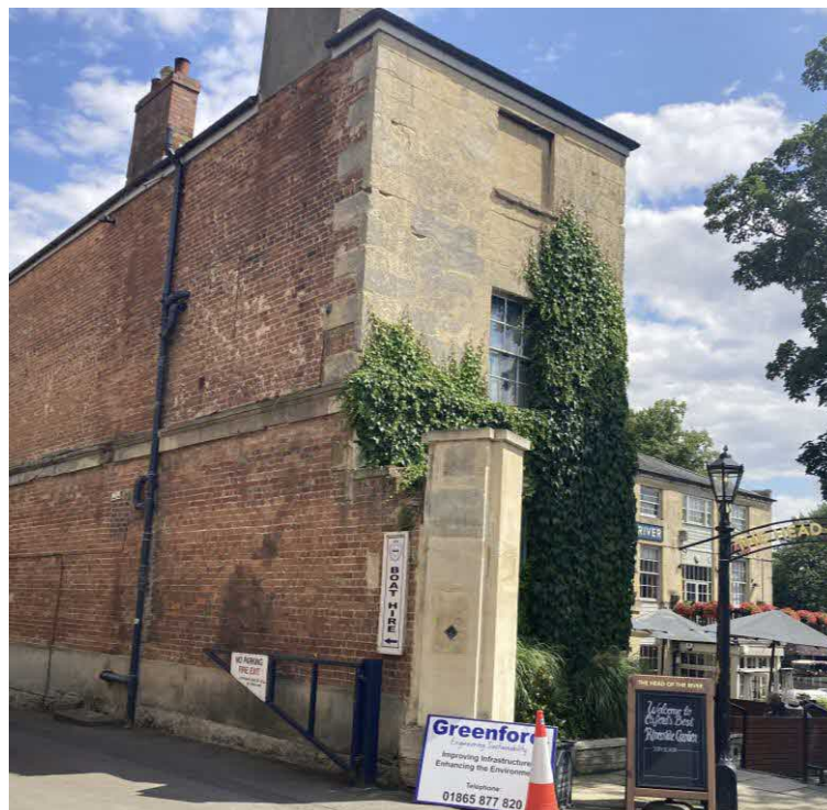
Above – Existing previously repaired stone pillar to front of Wharf House
