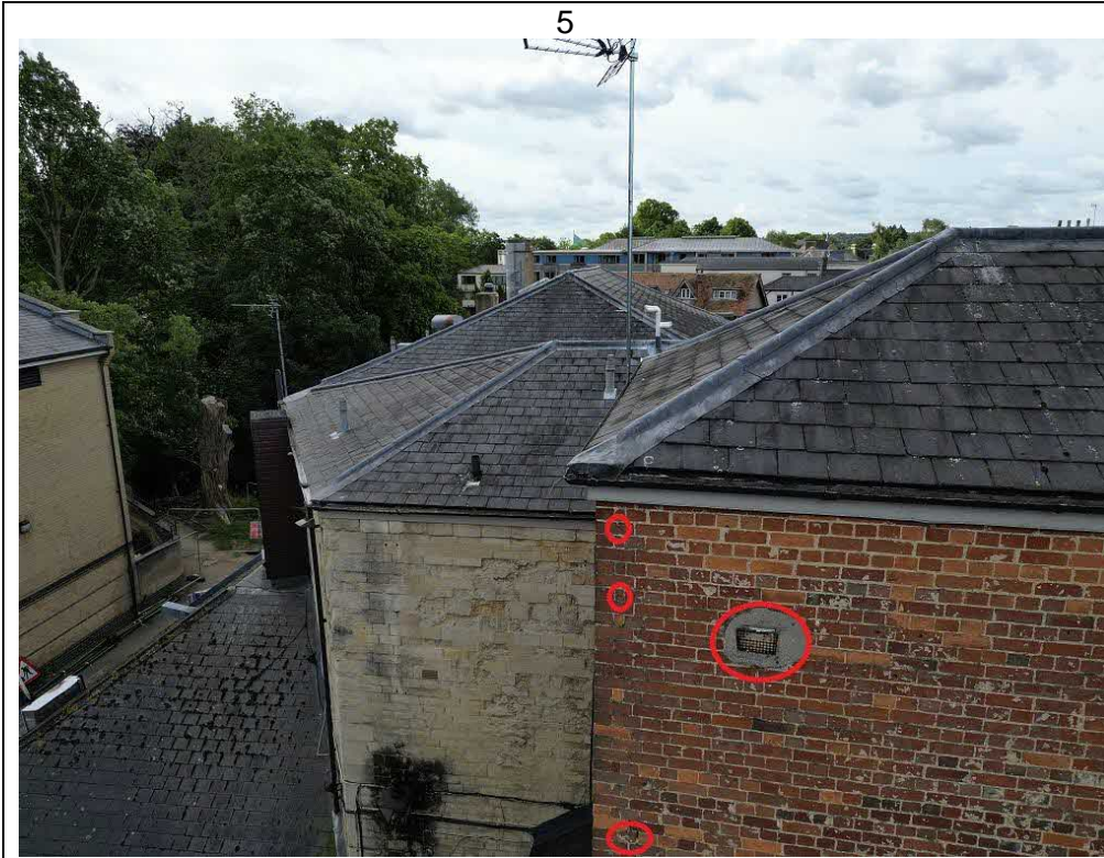
Spalling brickwork
