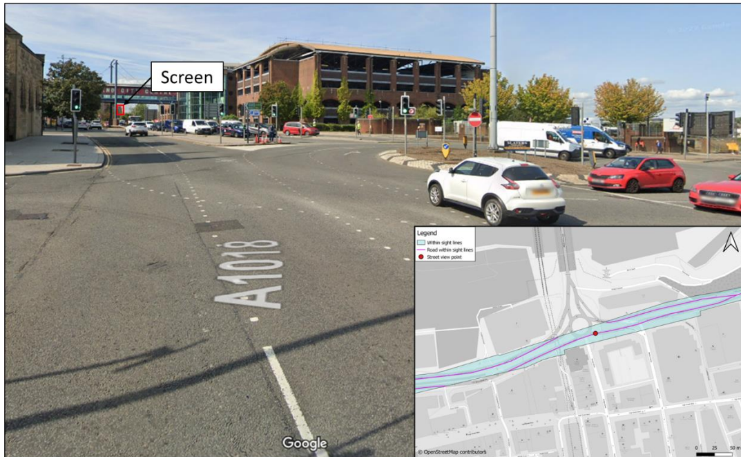
Figure 8. Eastern approach A1018/A183 roundabout (source: Google Maps)
