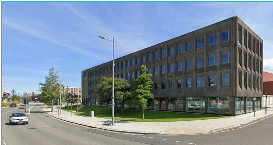
Figure 5.1 Former Gilbridge Police Station ('The Yard') in views from the A183
